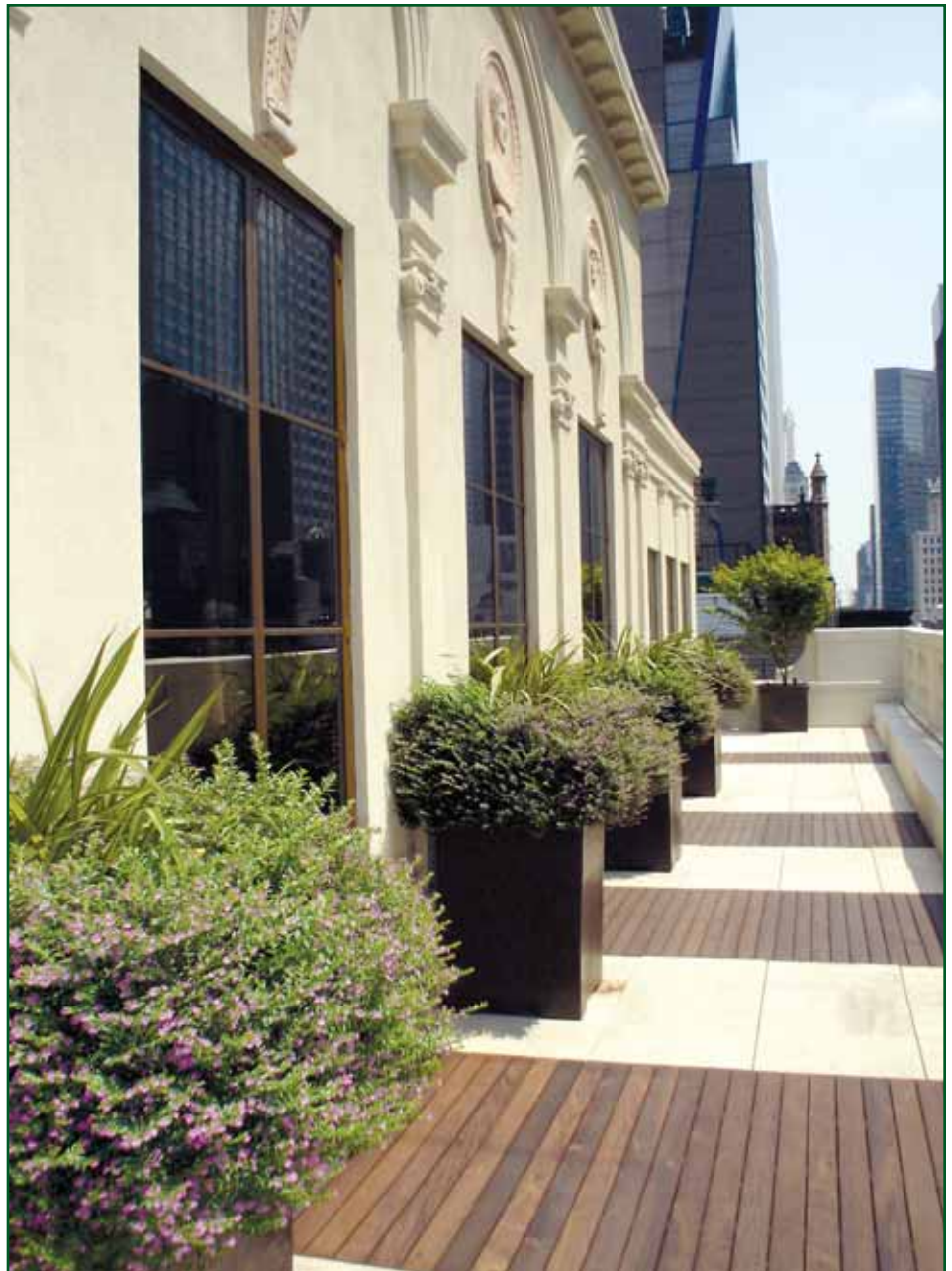
This large penthouse terrace was designed as an outdoor environment to complement a multi-million-dollar apartment high atop the New York City skyline, with multiple levels requiring exceptional waterproofing, especially around the flashings.
