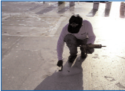
Photo 24 - Applying sealant to damaged areas on single-ply.
