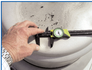
Photo 16 – Hole in barrel skylight.
