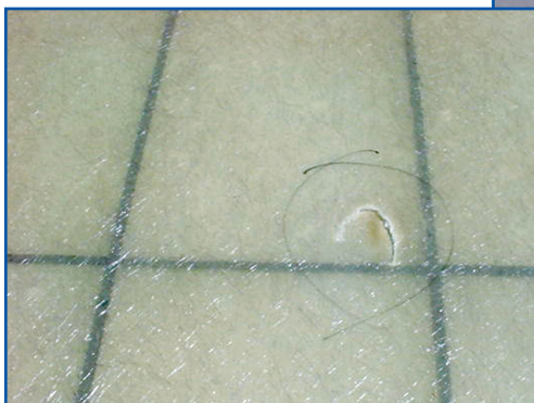
Photo 14 – Fracture in fiberglass skylight.
