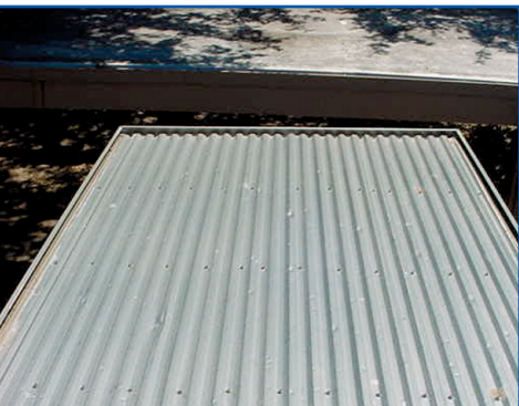
Photo 11 – Large dents in metal canopy.
