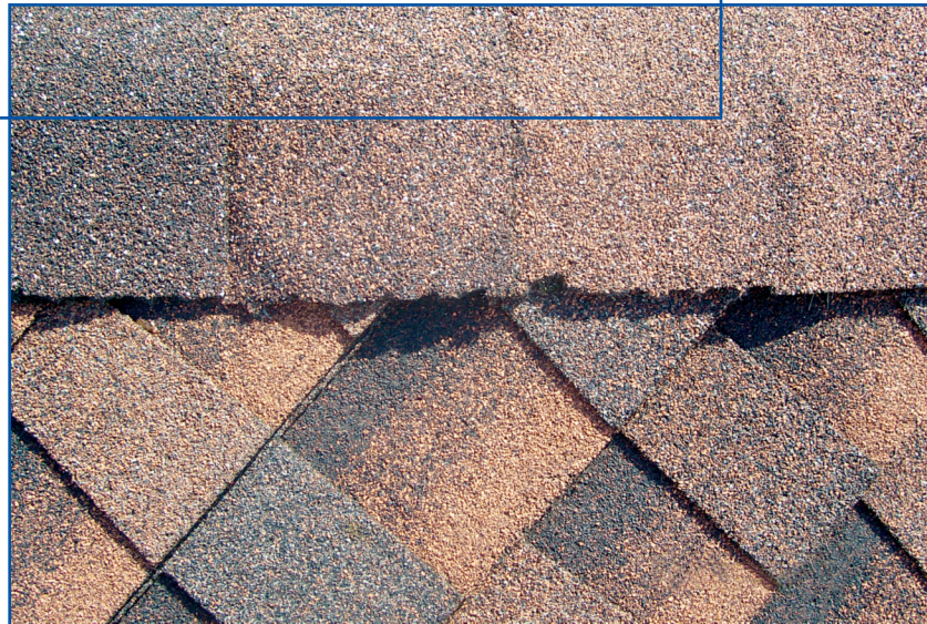
Photo 13 – Damage to edges of ridge shingles.
