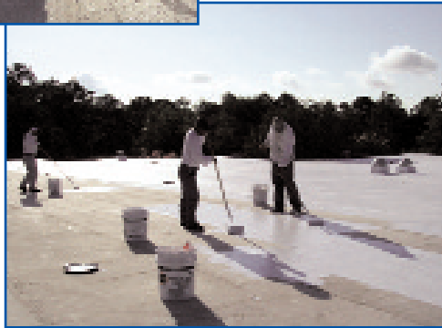
Photo 25 - Applying coating to damaged single-ply membrane.
