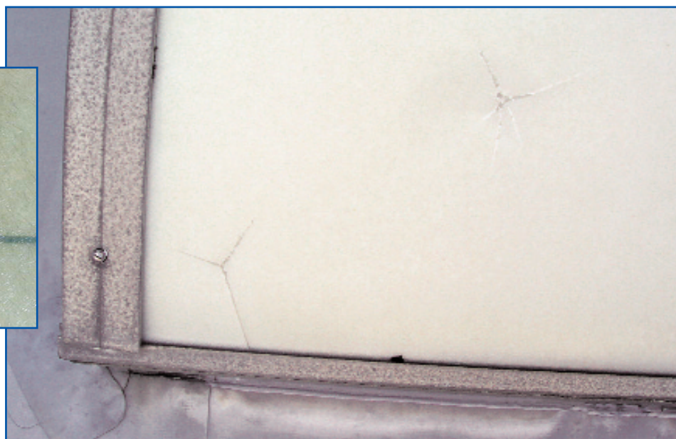
Photo 14 – Fracture in fiberglass skylight.
