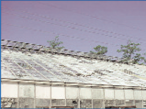
Photo 21 – Significant damage to glass panels.
