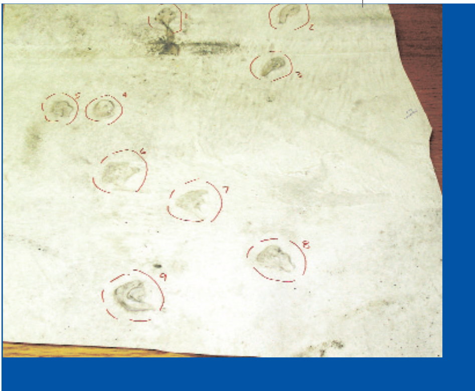
Photo 44 – Sealant and coating applied over membrane.
