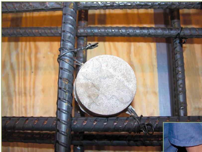
Figure 13 - Installation of an embedded sacrificial anode.
