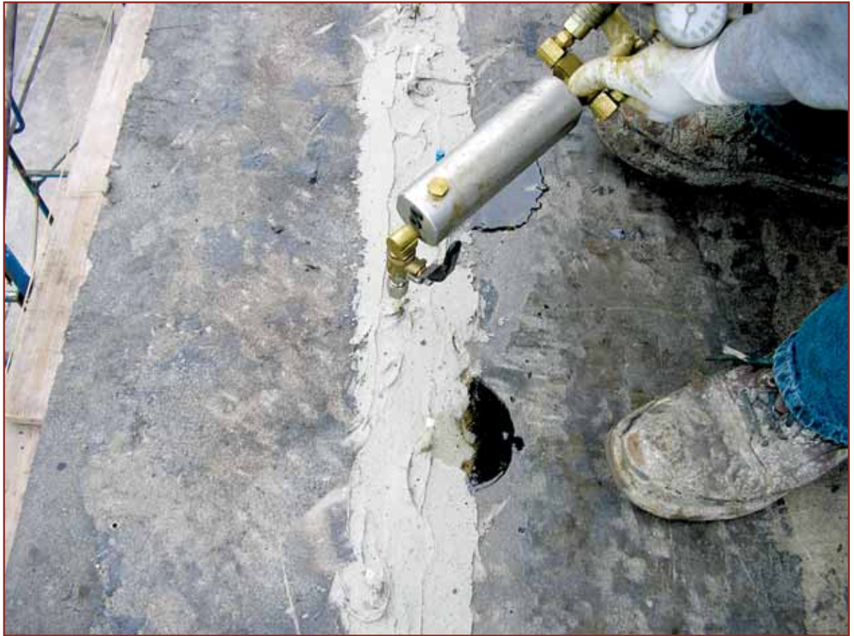
Photo 8 – Epoxy injection of a concrete slab
