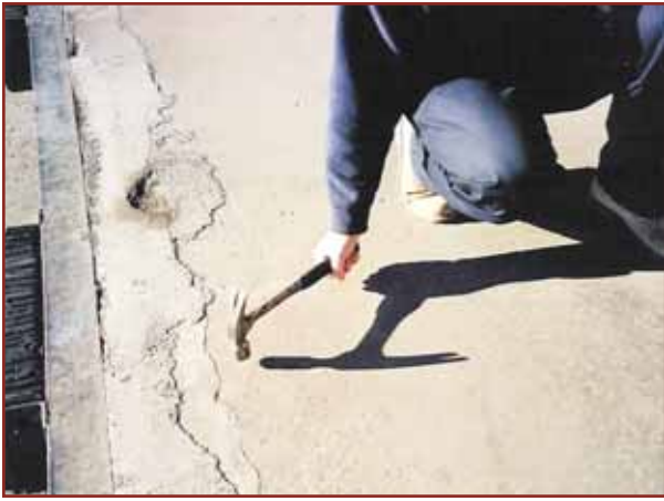
Photo 6 – Sounding of concrete by striking with a hammer
