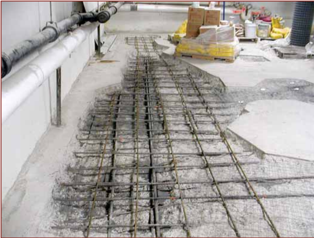
Photo 7 – Properly prepared surface repair
