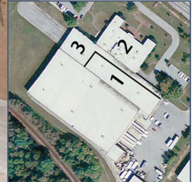
Figure 4 – Aerial view of the building identifies location of the roof areas shown in Figures 1, 2, and 3. The truck bay in figure 3 is numbered as 1; the area shown in Figures 1 and 2 is labeled 2; the number 3 is the area at the end of the truck bay that was not blown off. Satellite photograph courtesy of i-cubed ( www.i3.com ).
