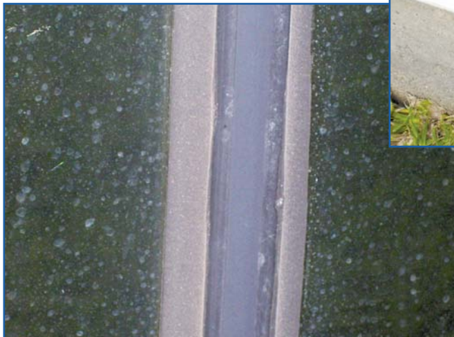
Figure 10 (below) – Wet seal applied along edge of gasket.
