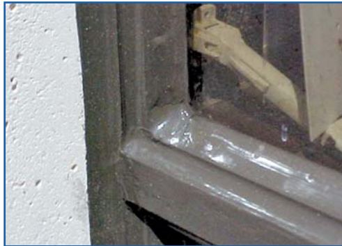
Figure 15 – Installed wet seal at window frame.
