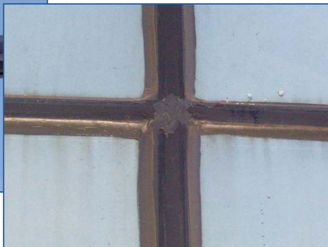
Figure 13 – Wet seal of lock-strip gasket.
