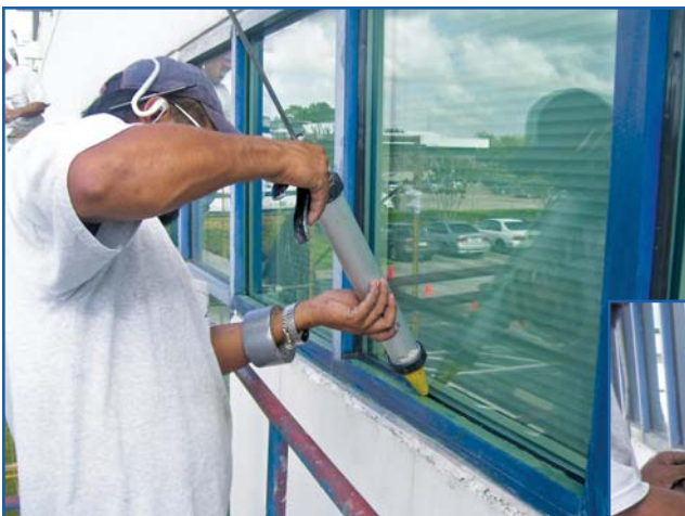
Figure 6 – Wet sealing window frame.
