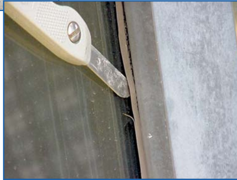
Figure 4 – Loose gasket.
