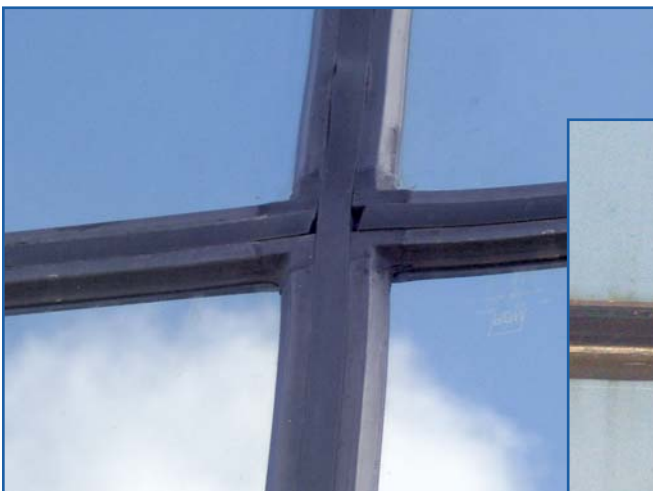
Figure 12 – Lock-strip gasket corner.
