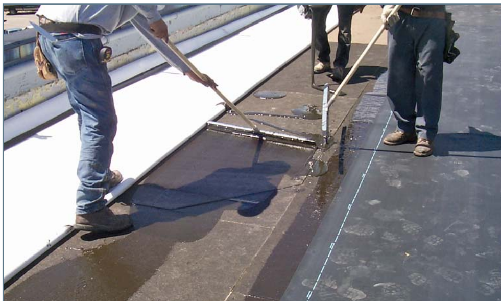
Photo 1 – High-solids, low-VOC, sheet-bonding adhesives can be applied easily with inexpensive equipment and minimal environmental impact.
