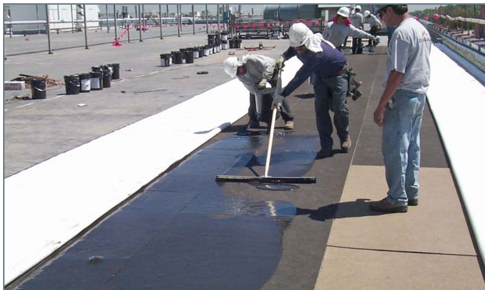
Photo 2 – Sheet-bonding adhesives can provide superior performance to mechanical fasteners while maintaining roof membrane integrity.
