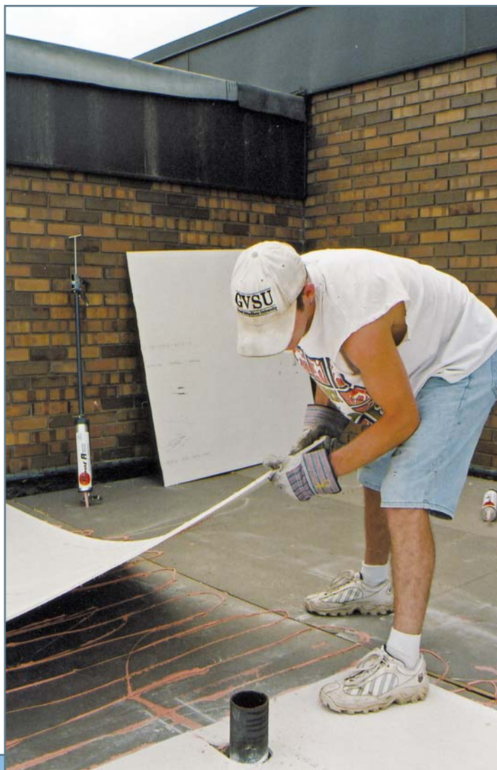
Photo 3 – New thermosetting foam and moisture-cure adhesives have been developed that will char before they melt, solving the fire-hazard problem.
