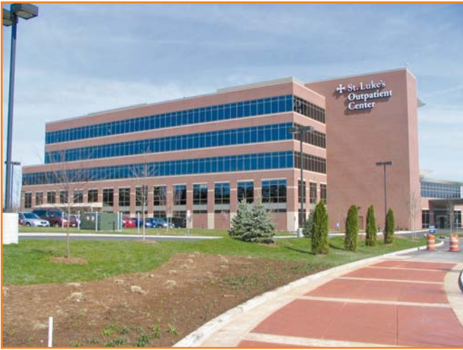
Photo 1 – Front of St. Luke's Outpatient Center.
