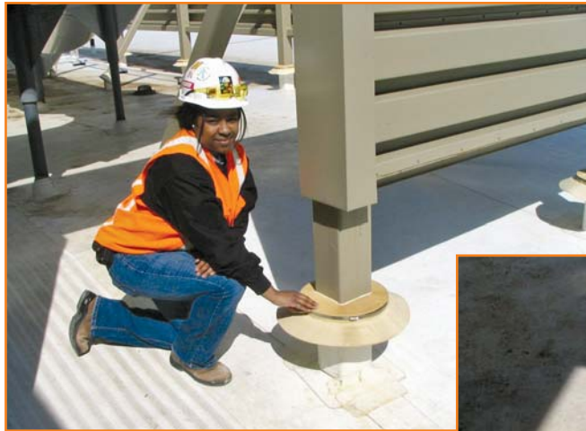
Photo 5 – Worker with 12-inch collar on equipment screen footer.
