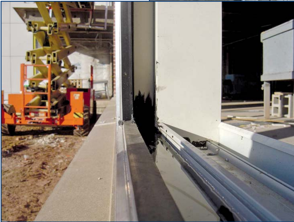
Photo 8 – This sill drainage test is being conducted without the glazing installed.
