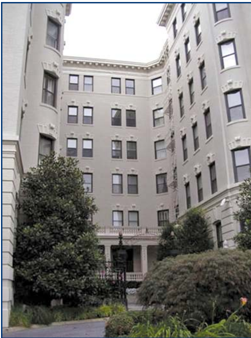
Photo 6 – This façade is a brick masonry mass wall assembly.
