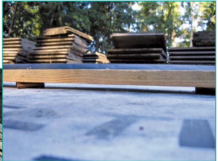
Figures 3A and 3B – Counter-batten (A, at left) or shimmed battens (B, above) improve ASV and drainage.
