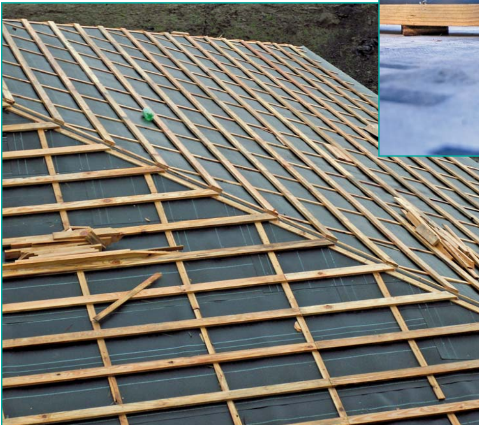
Figures 3A and 3B – Counter-batten (A, at left) or shimmed battens (B, above) improve ASV and drainage.
