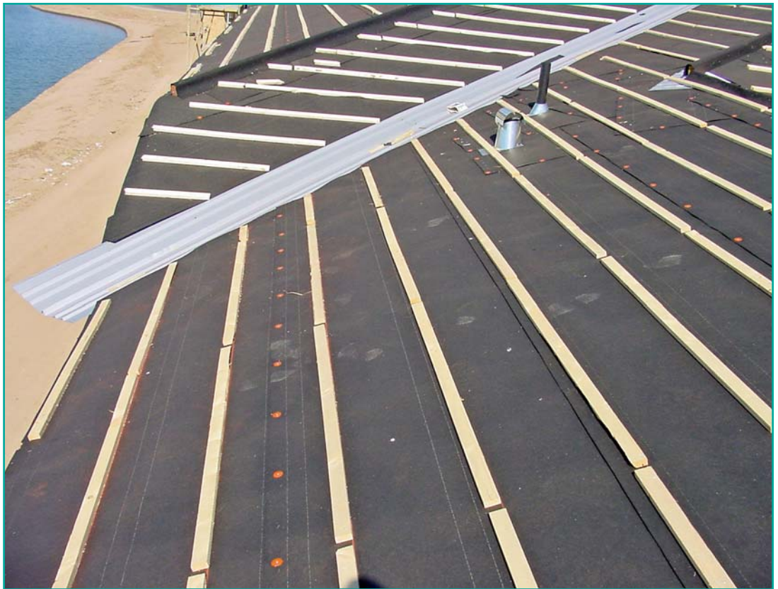
Figure 4 – Standard batten system.
