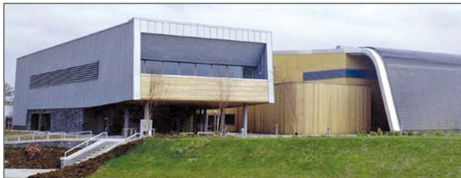
Figure 10 – The main elevation of OpTIC (Opto-electronics Technology and Incubation Centre), United Kingdom, showing the cantilevered business center and 1,000m 2 PV wall array.
