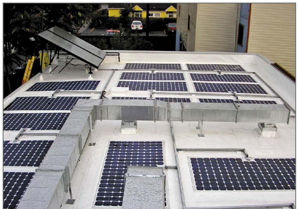
Figure 5 – Open Energy modules and single-ply membrane system.
