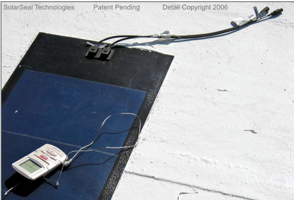
Figure 6 – SolarSeal System over SBS membrane with Uni-Solar PV module.
