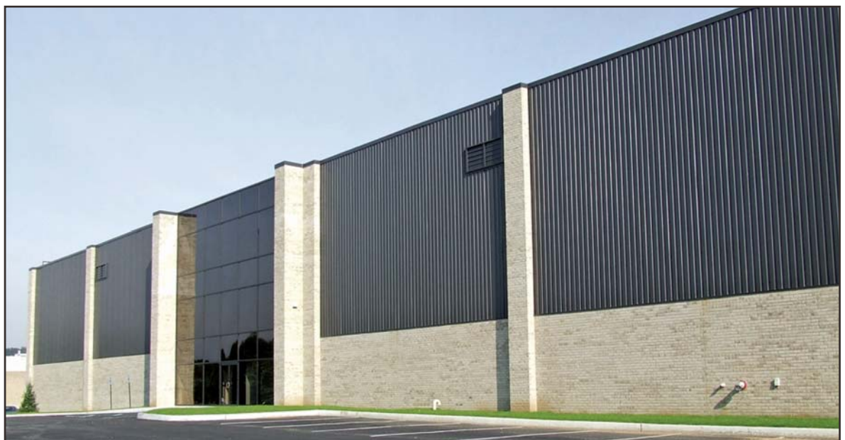
Completed installation of Grant Way Industrial building in Allentown, PA.
