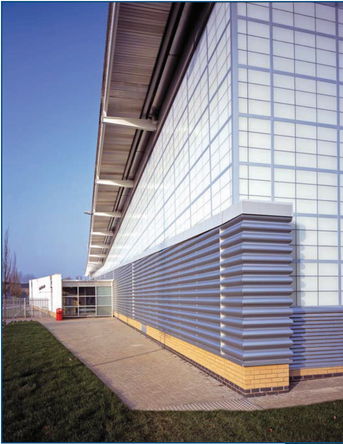
The Birmingham High-Performance Centre, Birmingham, England, features constant light levels that are enhanced by curtain walls. To prevent light pollution, the translucent curtain walls prevent direct-beam nighttime illumination from leaving the building site while creating a warm glow to the building exterior. (Photo by Adam Wilson and courtesy of Kalwall, Manchester, NH.)
