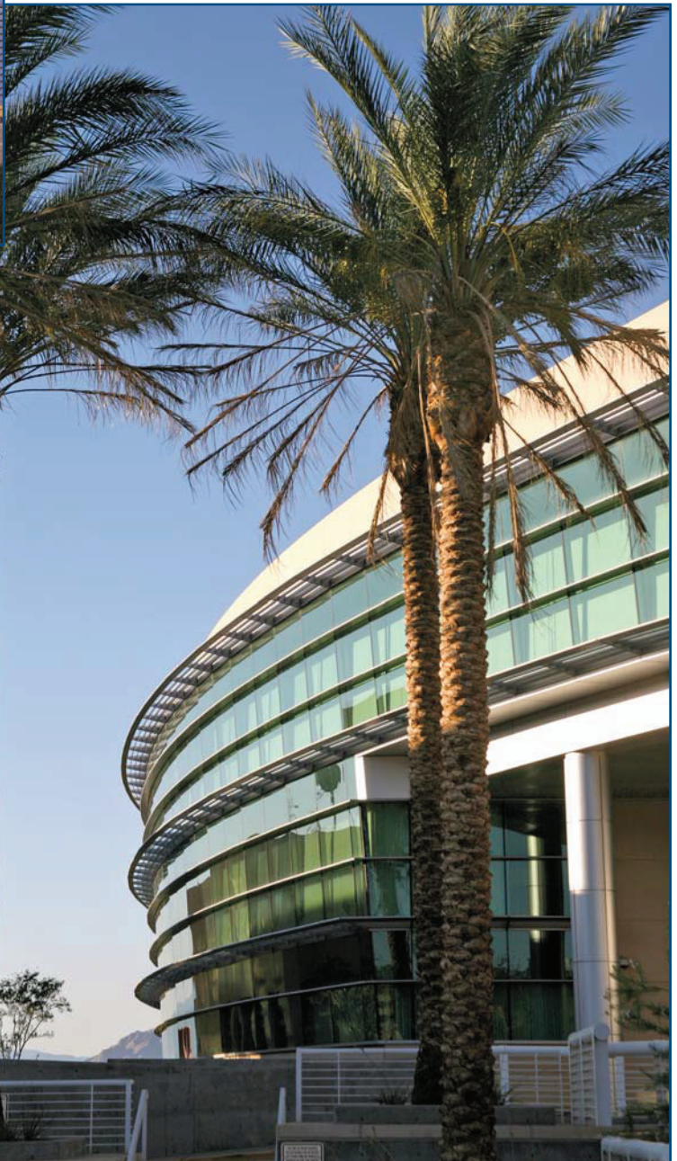
The City Hall Development Services Center, Henderson, NV, features curtain wall systems with a sun-shade product to minimize solar heat gain. (Photo provided by Vistawall, Terrell, TX.)
