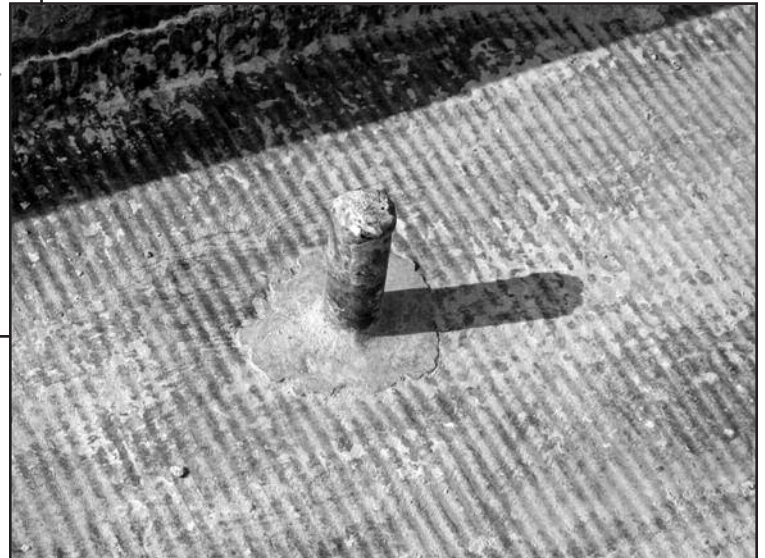
Figure 2 - Copper cup (thimble) from a circa-1930s project.
