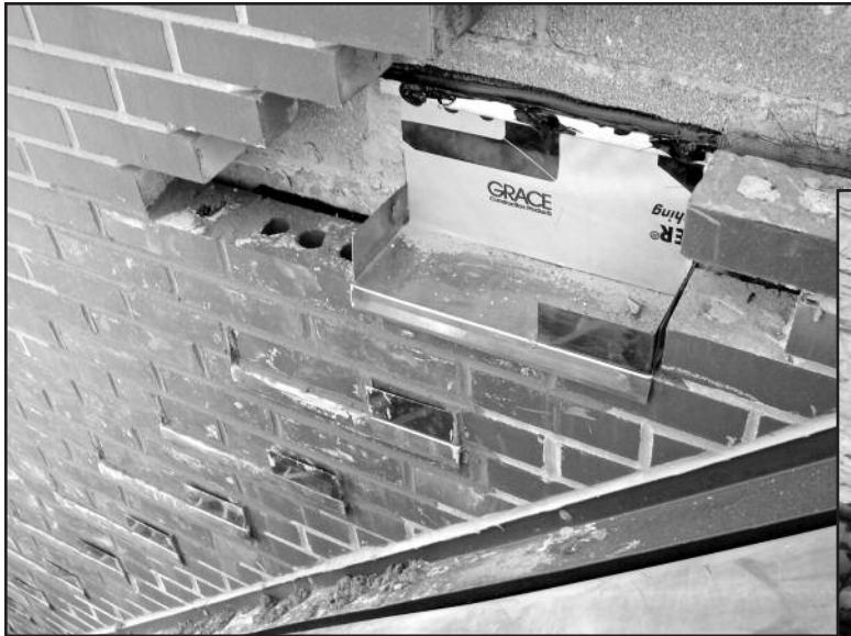
Figure 8 – Installation of copper stepped-pan flashing at raked rising wall.
