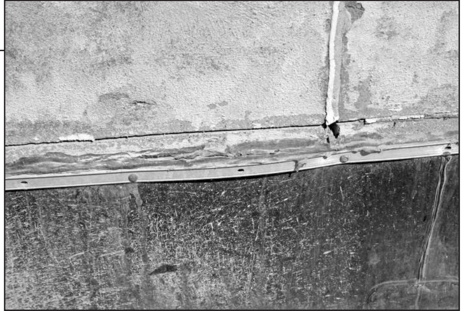
Figure 5 – EPDM roof membrane terminated at cast stone parapet.
