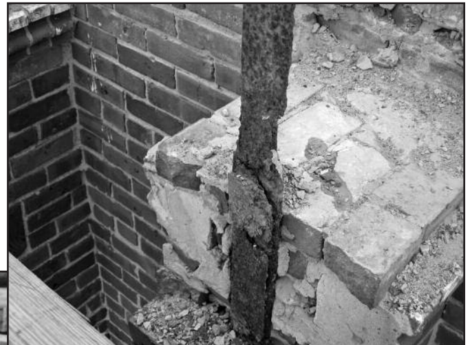
Figures 10a (left) and 10b (above) – Displaced brick masonry caused by oxide jacking of embedded steel hangers.
