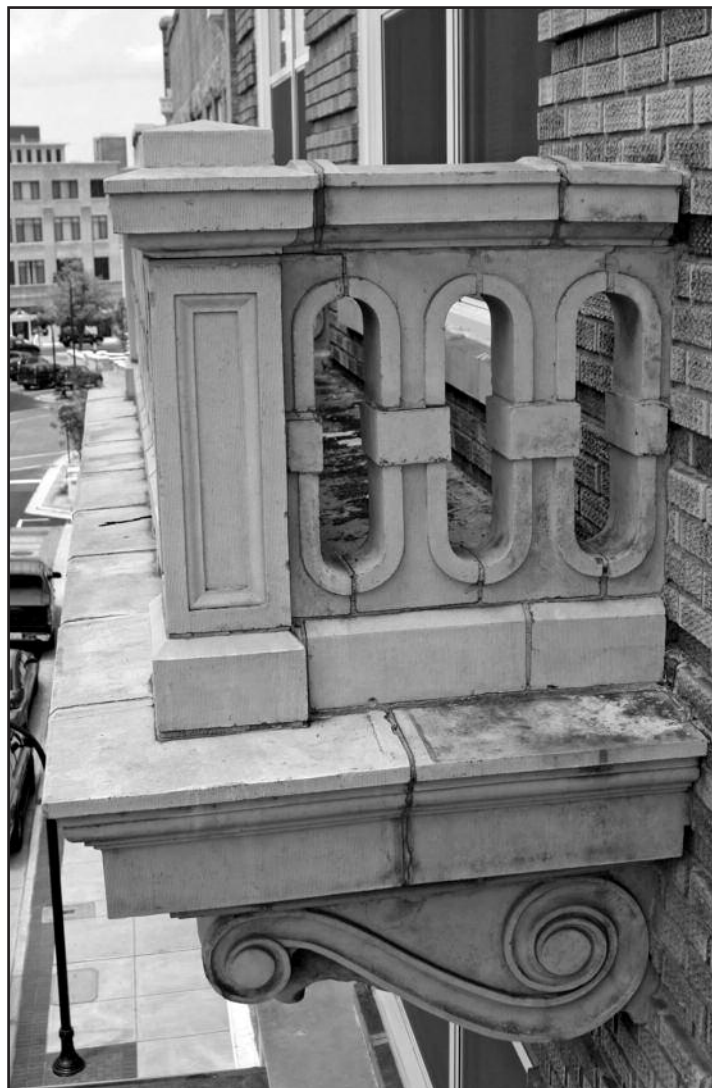
Figure 13 – Terra cotta balcony assembly.
