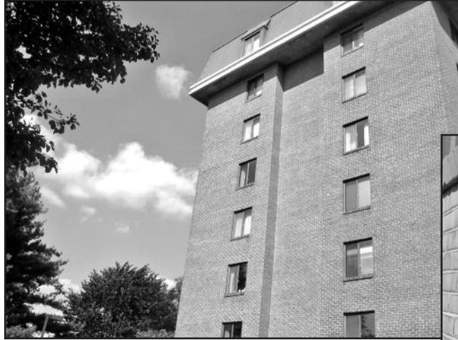
Photo 1 - Multistory brick-masonry-clad building with punched windows.
