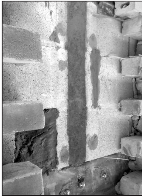
Photo 11 – Installation of grout around steel reinforcement in concrete masonry backup wall.
