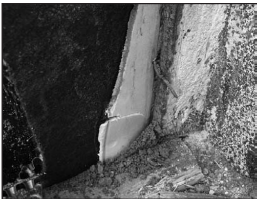
Void between soldier pile and foam protection board was also evident and may have contributed to the failure of the bentonite waterproofing system.
