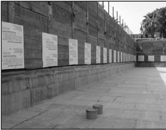
Conventional wood lagging.
