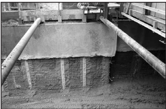
Void behind foam protection board, shotcrete lagging.
