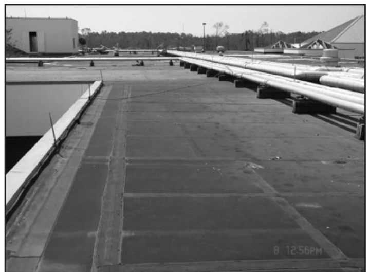
Figure 10 – This perimeter fastening is designed for high wind resistance. (Photo courtesy of RICOWI Inc.)
