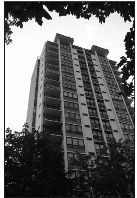
Photo 4 - This 24-story reinforced concrete high-rise had floor-to-ceiling window/spandrel panel assemblies and concrete shear walls.
