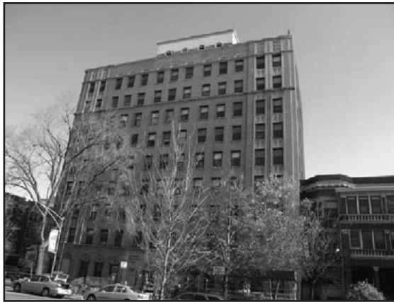
Photo 1 – This circa 1920 building has a reinforced concrete structural frame and masonry/terra cotta façade supported with steel shelf angles.
