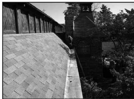
Figure 3 – The outside edge of these built-in gutters is set too low. In a heavy downpour, rainwater can overshoot the gutters and run down the exterior masonry walls.
