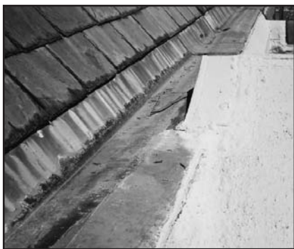
Figure 3 – The outside edge of these built-in gutters is set too low. In a heavy downpour, rainwater can overshoot the gutters and run down the exterior masonry walls.
