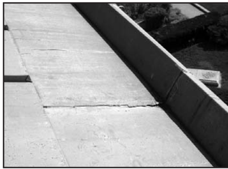
Figure 1 – Open seam (left) and fatigue crack (right) in two different lead-coated copper gutter liners. Both are due to lack of expansion joints to accommodate thermal movement in the gutter liners.
