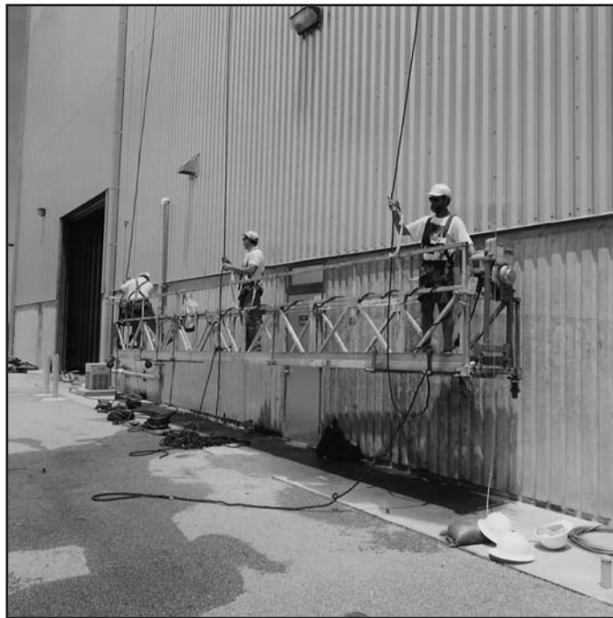
Figure 1 – Inspection of wall using swing staging.
