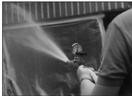
Figure 3 – Water spray test used to locate source of leak.
