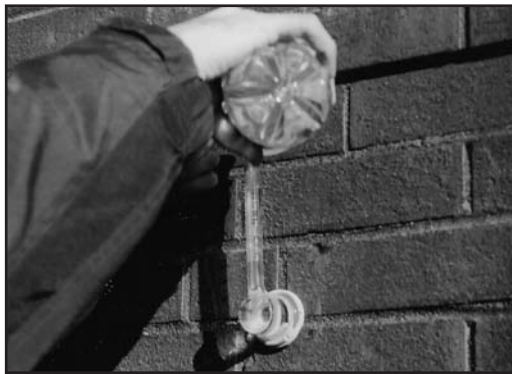
Figure 2 – Performing a RILEM tube test to determine porosity of a masonry wall.
