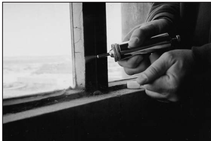
Figure 6 – Using a smoke/dust tracer to find air infiltration.
