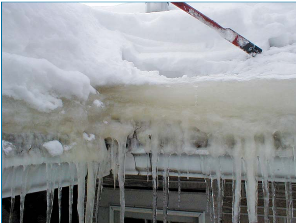
Ice dams can be more than 2 ft thick.
