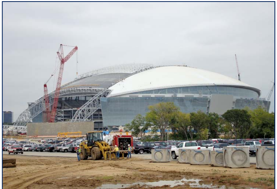
Figure 7 – Cowboys Stadium retractable roof and operable end-zone walls being constructed.
