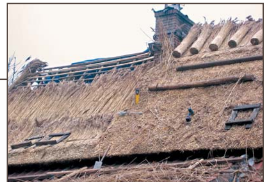
Rethatching in progress, Holland, 2006. Photo by Rasbak, Wikimedia Commons.
