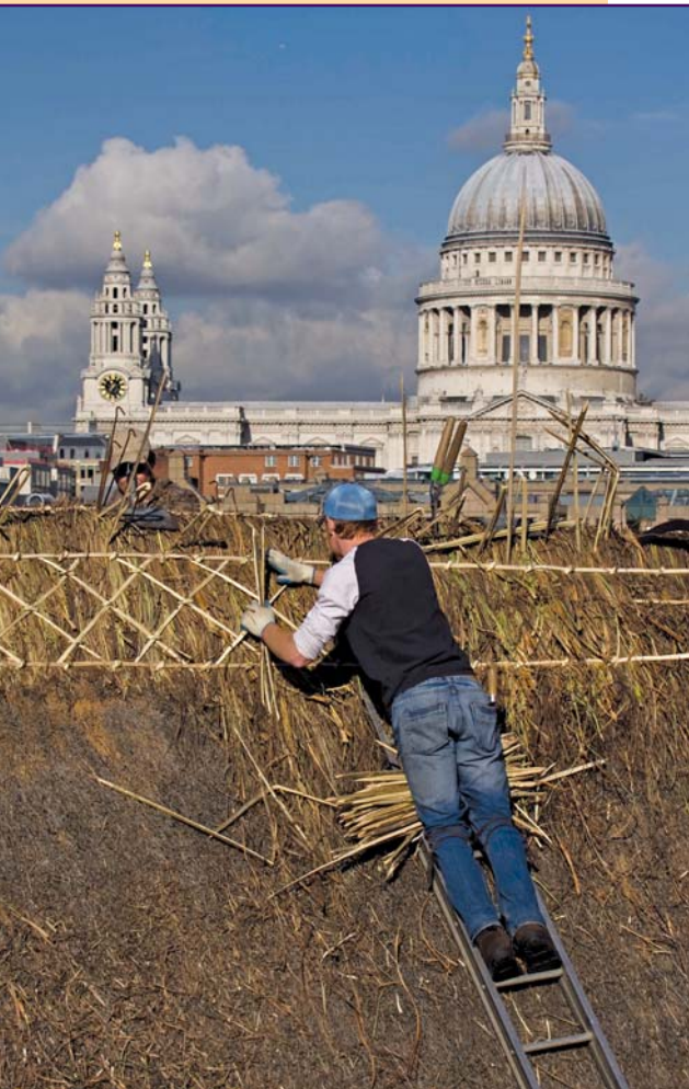
Thatcher pegging down the new ridge with hazel spars. Photo © Nathan Harrison.
