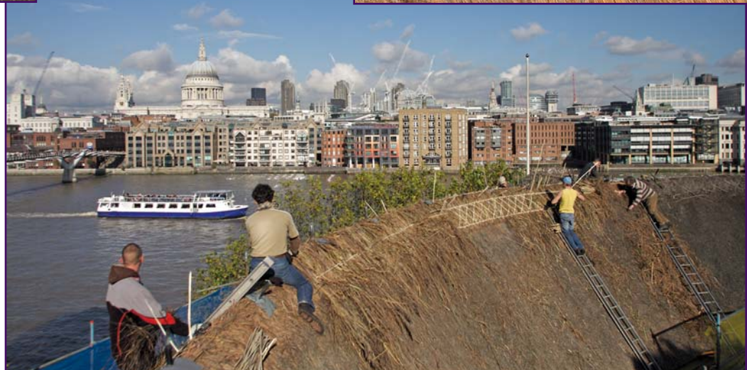
Thatcher pegging down the new ridge with hazel spars. Photo © Nathan Harrison.
