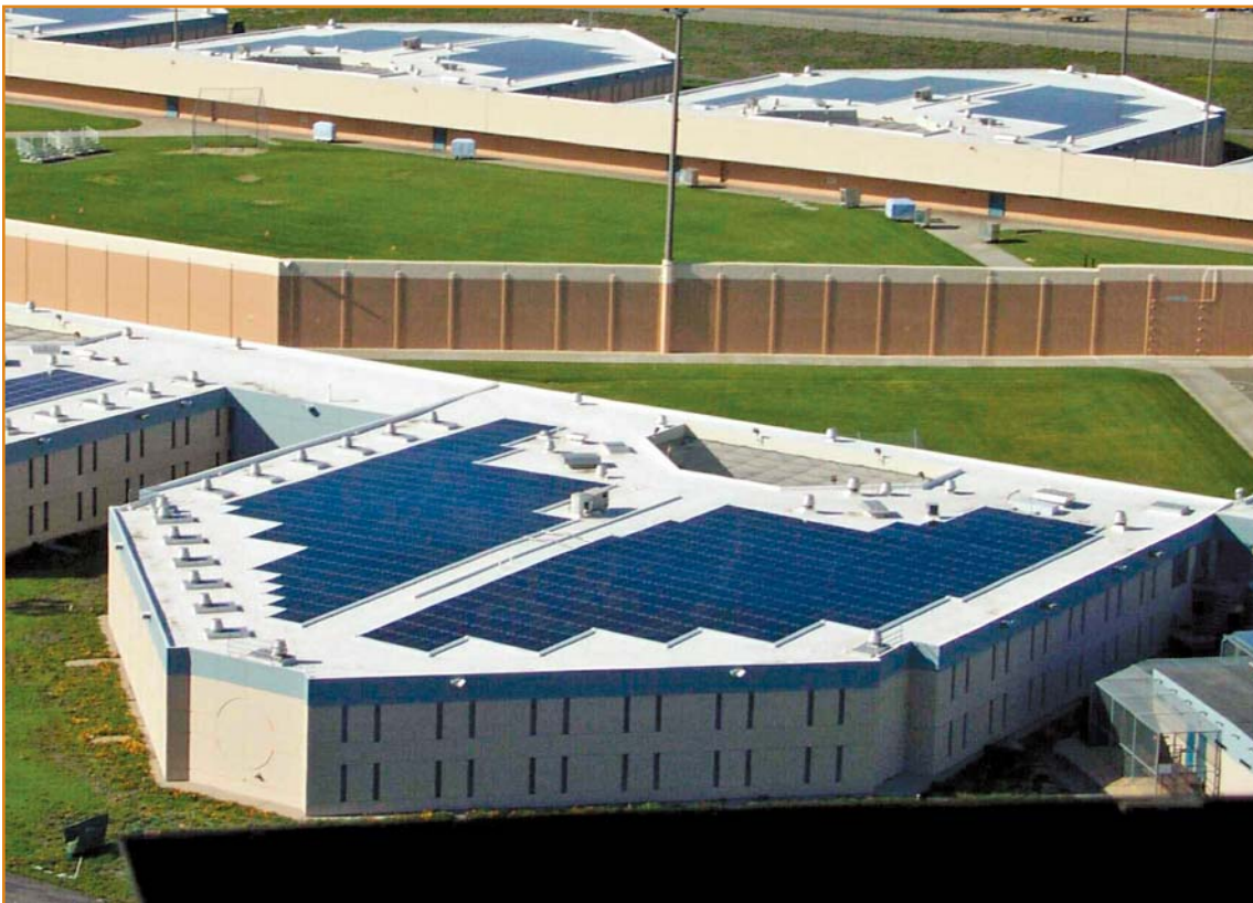
Photo 2 – Many roof designers are excited about the potential of vegetative and photovoltaic (PV) roofing systems. However, construction-related moisture problems are common to all types of roofs. (Photo courtesy of GAF Materials Corporation, Wayne, NJ.)
