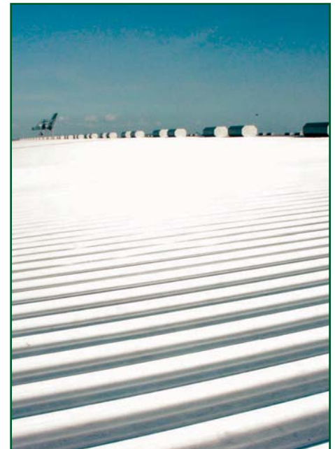
Figure 4 – Concealed fastened panels eliminate most fasteners from the weathering surface by using hold-down clips inside the side-seam joint. The clips permit thermal movement, but because the “flat” of the panel is unrestrained, wind resistance is diminished. Under load, the panel flat arcs upward, rotating the seam and disjoining.
