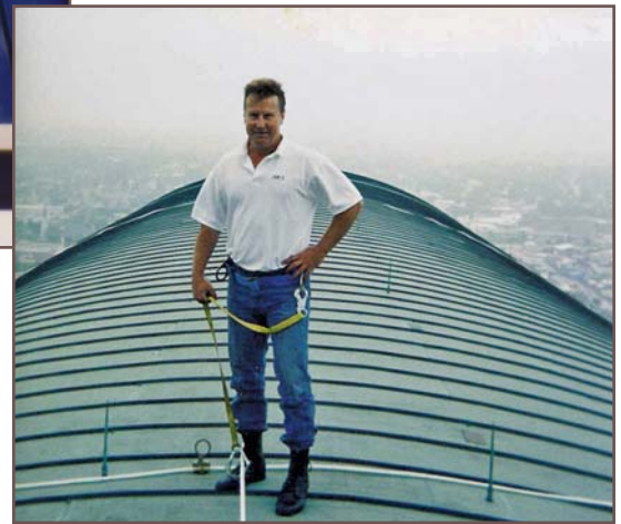
Figure 3 – The author (years ago) atop a curved copper roof having no ridge interruption (the nature of safety gear shown can probably date the image). This roof continues to serve satisfactorily on a corporate headquarters facility.
