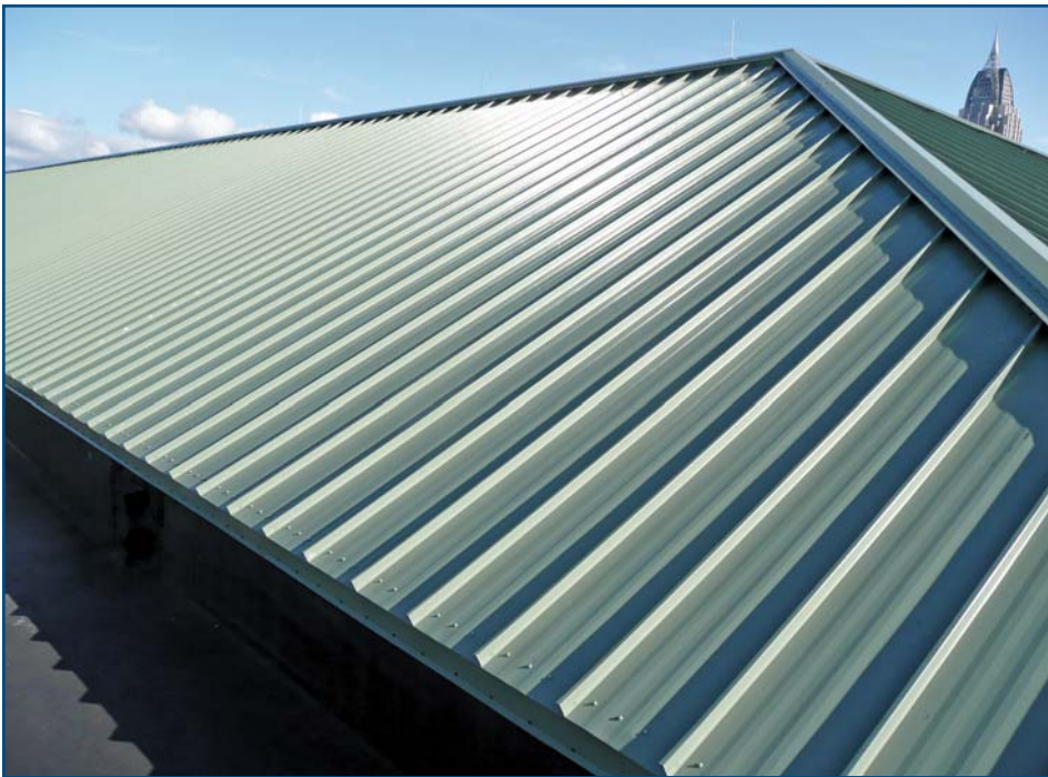
Photo 5 – Finished painted metal roof in coastal Alabama.
