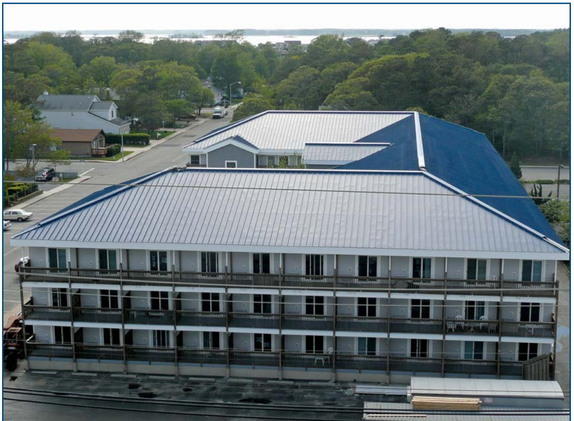
Photo 1 – Retrofit metal roof on a condominium located in Ocean City, Maryland.
