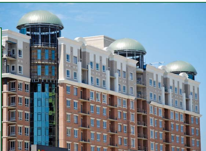
Photo 4 - All three domes in position.
