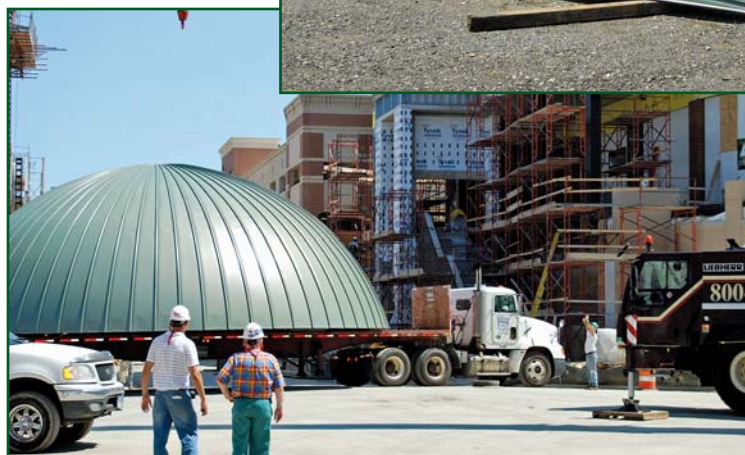
Photo 1 - Domes ready to be loaded at Lancaster Domes.
