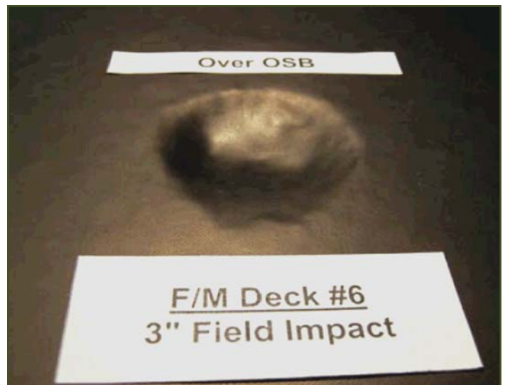
Figure 4 – Three-inch hailstone impacting EPDM membrane, tested over OSB. To obtain a copy of the full report on Koontz’s research, visit www.epdmroofs.org . (Photo courtesy of Jim D. Koontz and Associates Inc.)
