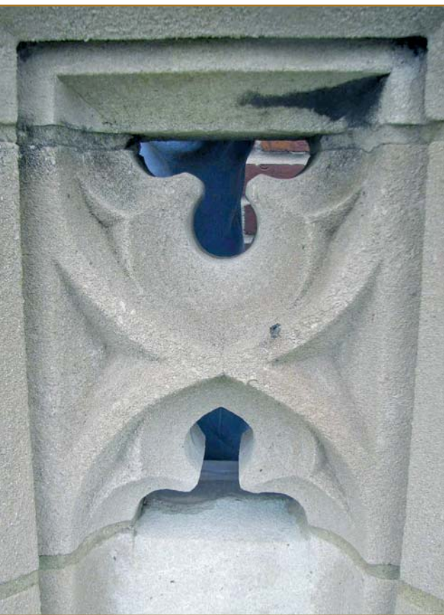
Photo 10 – Carved stone central to the three-stone set establishing the portal openings.
