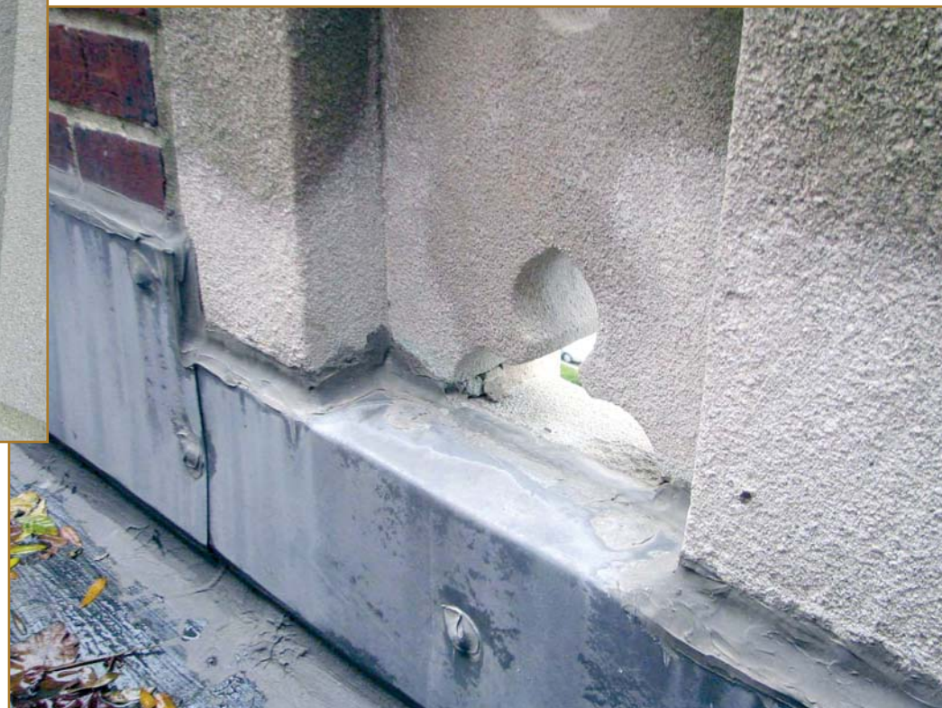
Photo 11 – Area of stone infill on roof side of parapet wall required to accommodate revised height of finished gallery roof.
