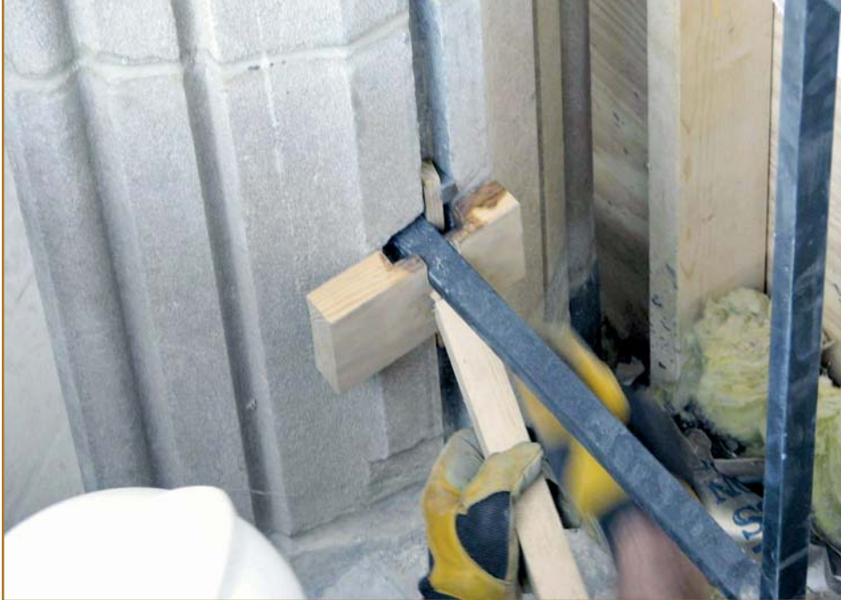
Photo 13 – Wood forms set in advance of pouring molten lead to fill the pocket in the stone surround.
