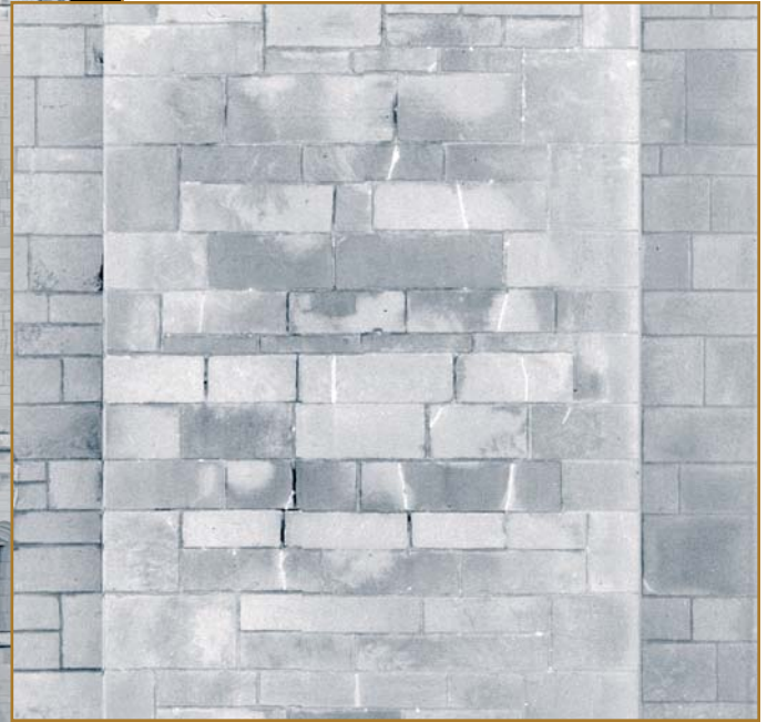
Photo 7 – Enlarged area of localized distress below tower balcony roof with failed drain leader.
