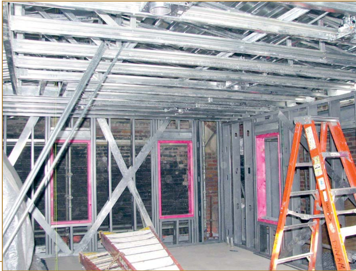
Photo 22 – New wall framing and truss assembly for the playing cabin.
