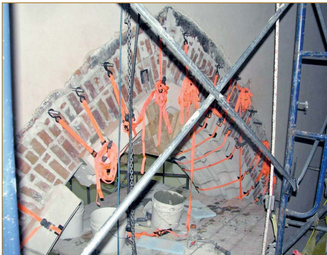
Photo 17 – Final setting of cut limestone surround in tonal opening.
