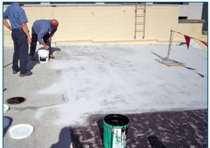
Broadcasting ceramic granule surfacing into cold-process adhesive.
