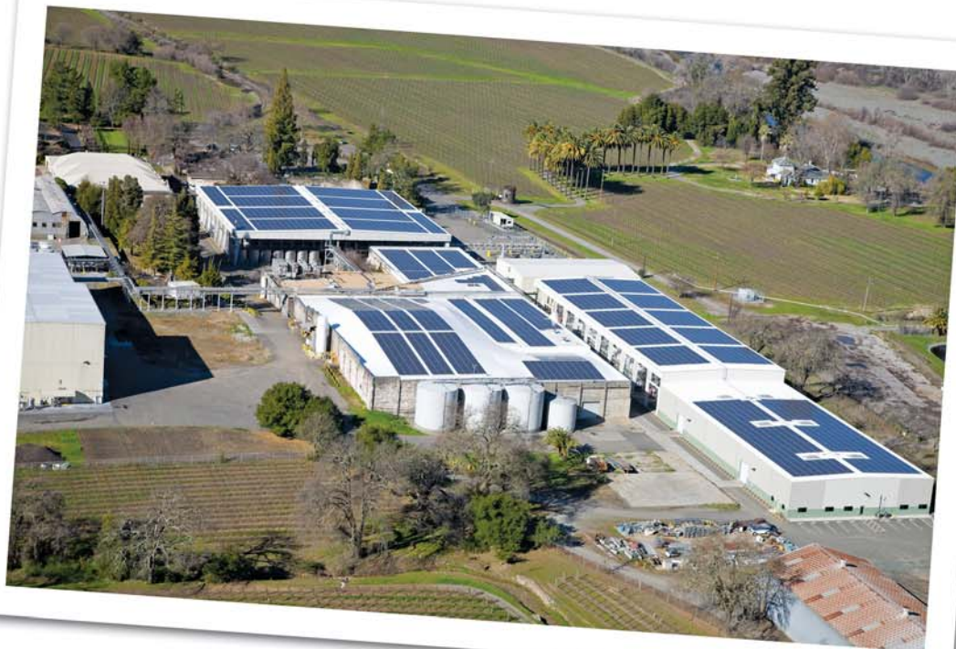
Aerial view of the solar installation at Asti Winery in Cloverdale, CA.
