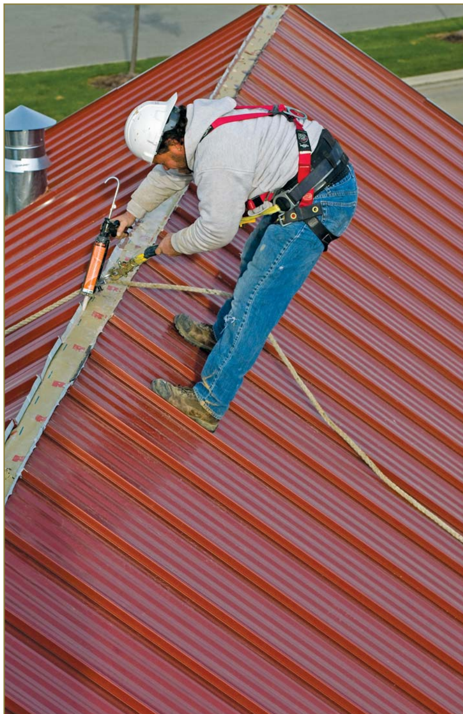
Worker on top of a metal roof.
