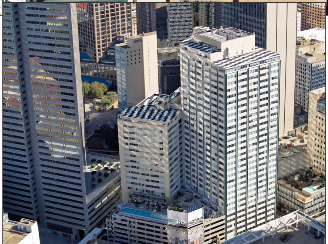
This downtown Dallas building was renovated into luxury condos. The developers wanted it to be seen by the high-rise buildings around it. Construction: Iso set in OlyBond 500, Liberty SA, SBS heat-weld 25, SBS heat-weld FR seen as white, Torch Plus FR seen as black.
