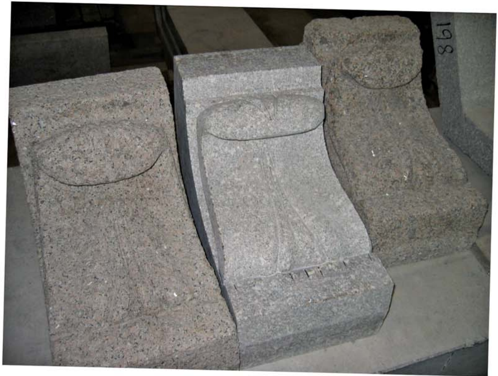
Figure 21 – Existing and new granite bracket during fabrication.
