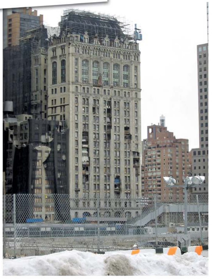
Figure 6 – North façade as the building looked after initial cleaning, after removal of loose materials, and before the mast-climbing scaffold was installed.
