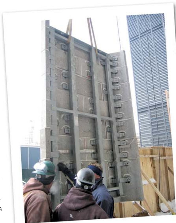
Figures 22A and 22B – New steel tube panels with stone facing installation.
