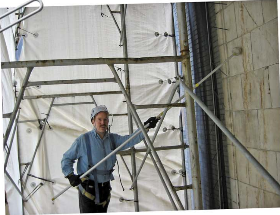
Figure 8 – Mark Anderson sounds terra cotta with a “sounding ball” at the north elevation.
