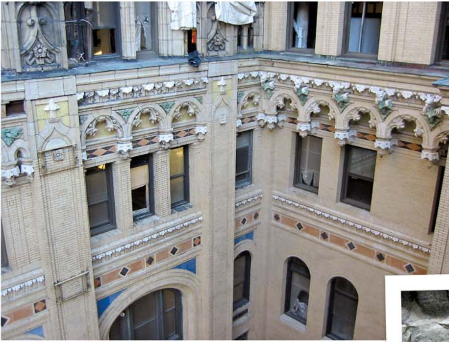
Figure 9C – Courtyard after cleaning, November 2003.
