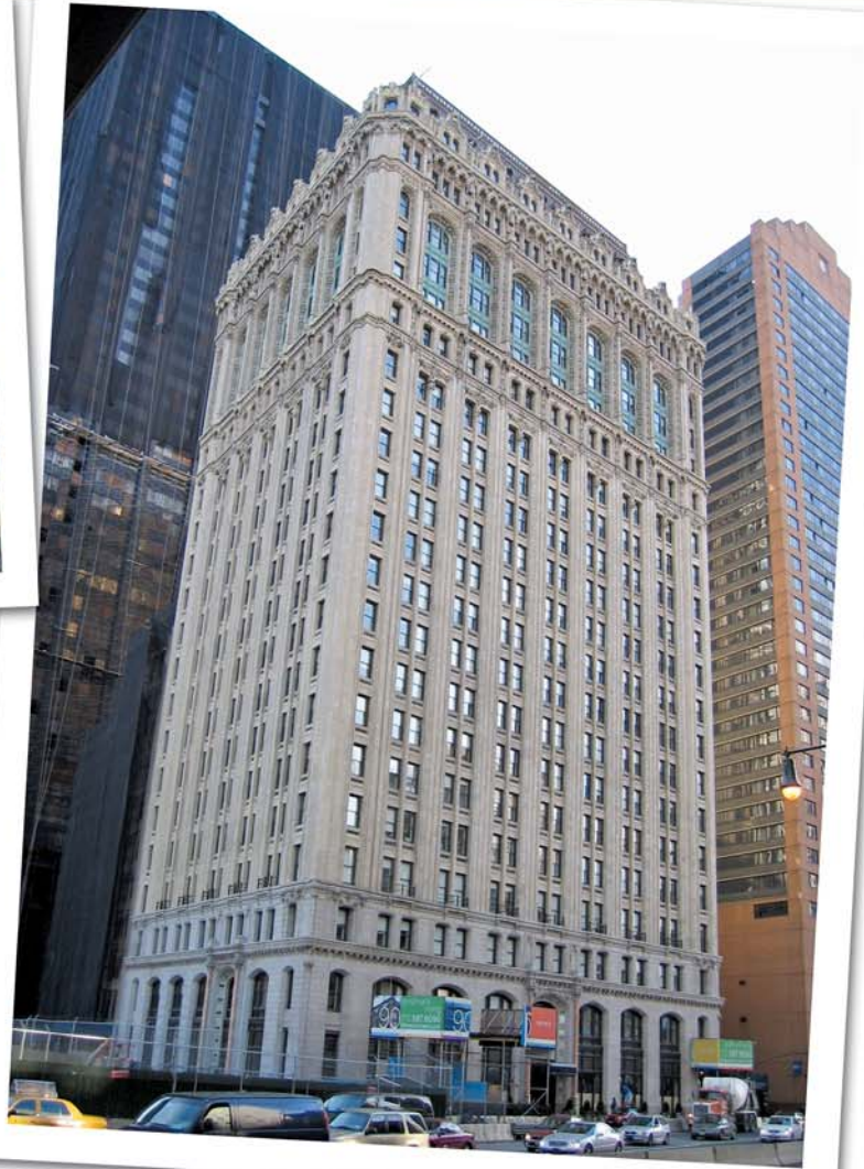
Figure 12 – Completed restoration at north and west elevations.
