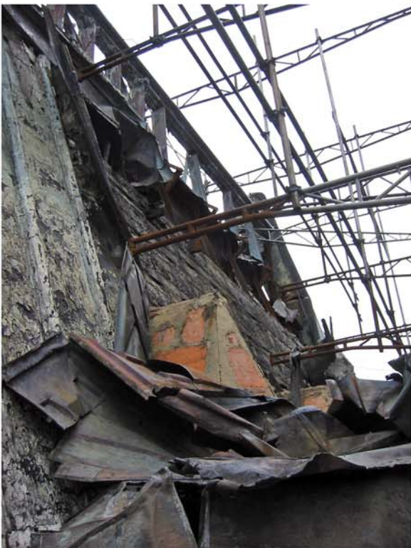
Figures 13A and 13B – Copper sheets on the mansard roof melted, and wood nailers burned from the fire on 9/11.
