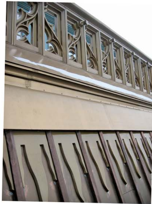
Figure 15B – Completed mansard roof with new fiberglass balustrade and icicles.
