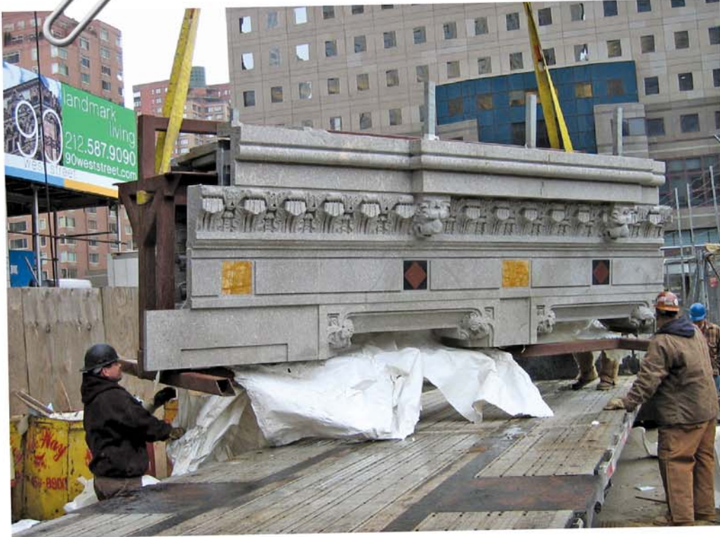
Figure 23 – Granite panel hoisted from flatbed truck.
