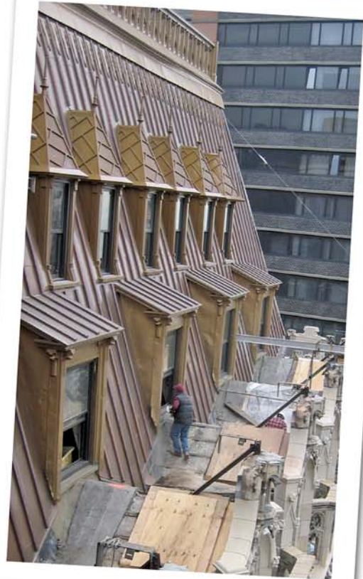
Figures 16A and 16B – West mansard roof before and after restoration.
