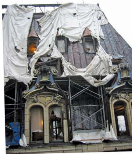
Figures 13A and 13B – Copper sheets on the mansard roof melted, and wood nailers burned from the fire on 9/11.
