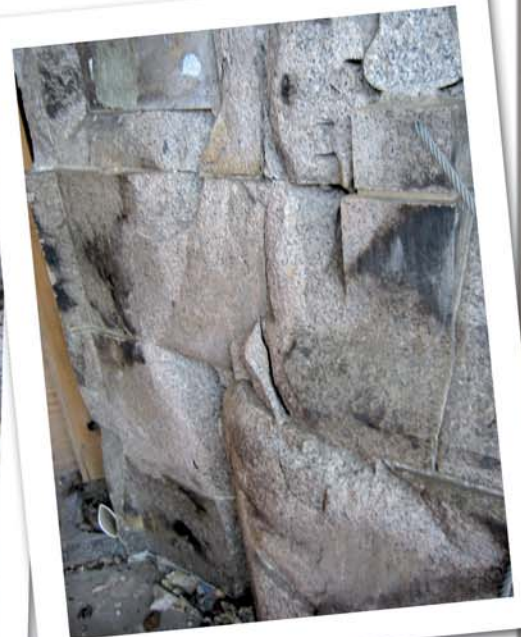
Figures 17A and 17B – Fire and impact damage rendered much of the north granite base unrestorable.
