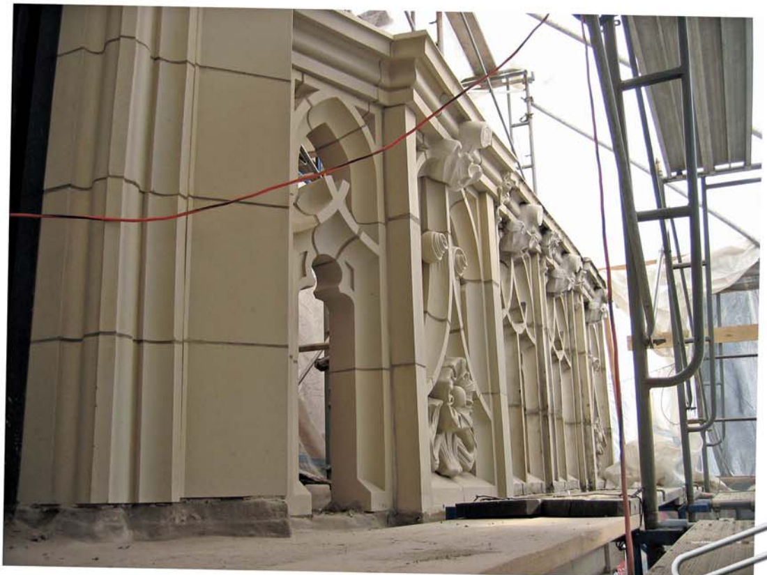
Figure 10 - New and existing terra cotta stones at screen walls.
