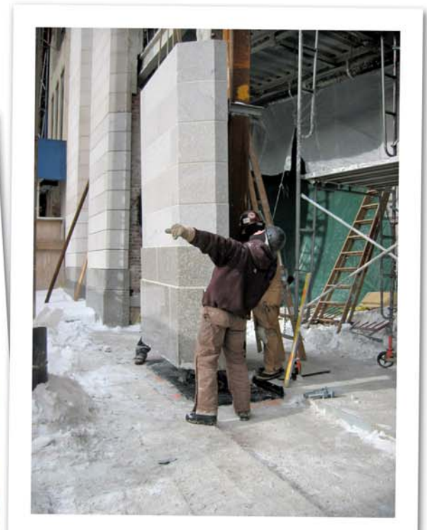
Figures 22A and 22B – New steel tube panels with stone facing installation.
