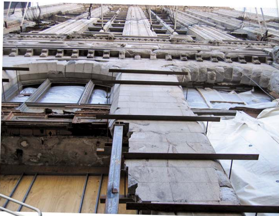
Figures 17A and 17B – Fire and impact damage rendered much of the north granite base unrestorable.
