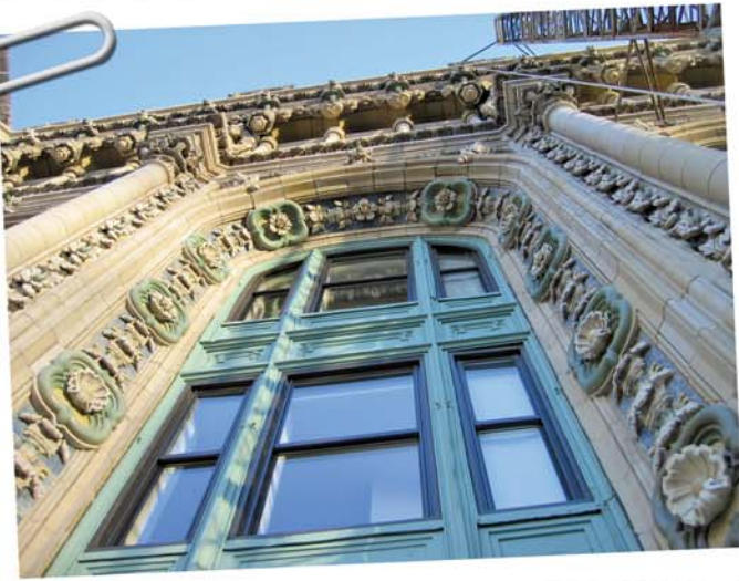
Figure 11 – Completed restoration of devastated area at top of north elevation.
