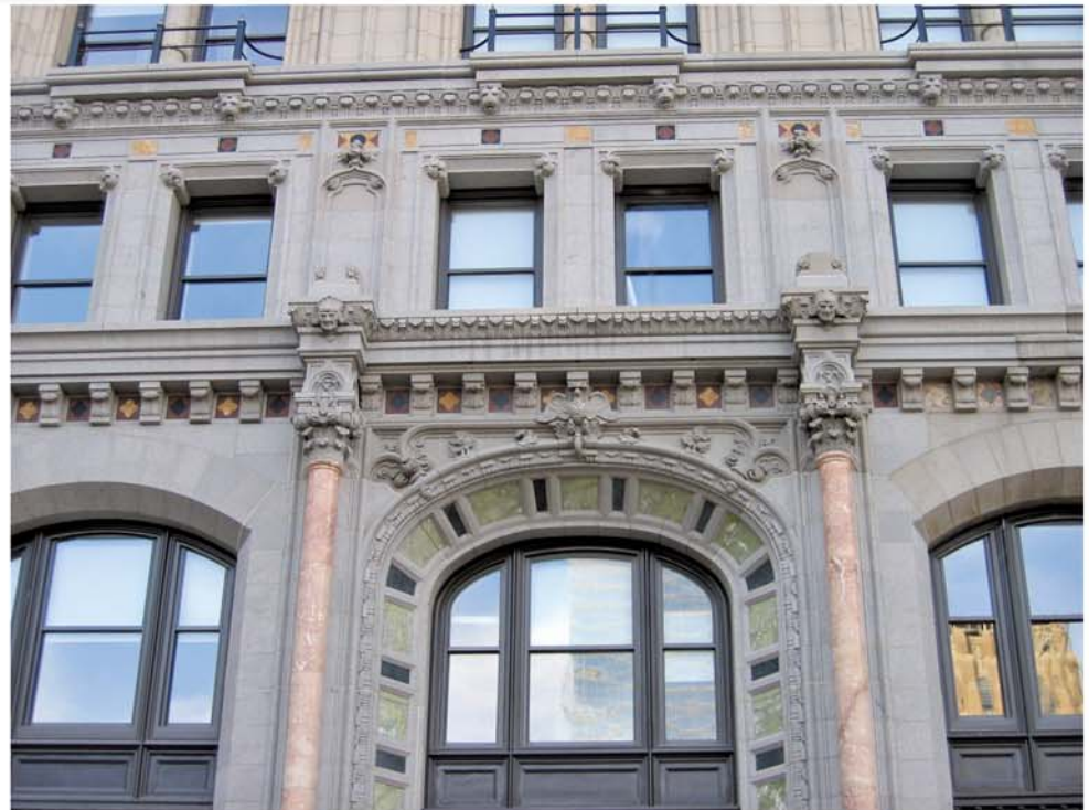
Figure 24 – Completed north entrance arch, December 2005, where approximately 50% of the original granite was reinstalled after being refitted onto the new panels. Compare with Figure 17A.
