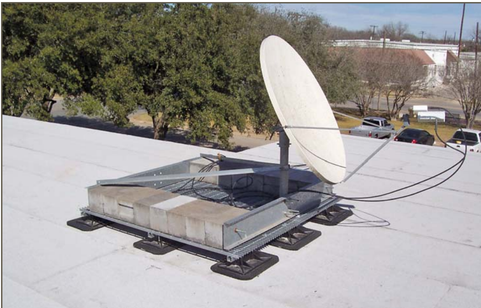
Figure 14 – Satellite dish installed on premanufactured support.
