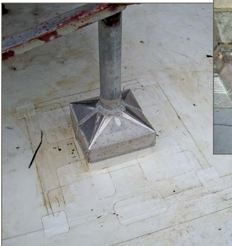
Figure 6 – Sheet metal pan and bonnet installed at round post.
