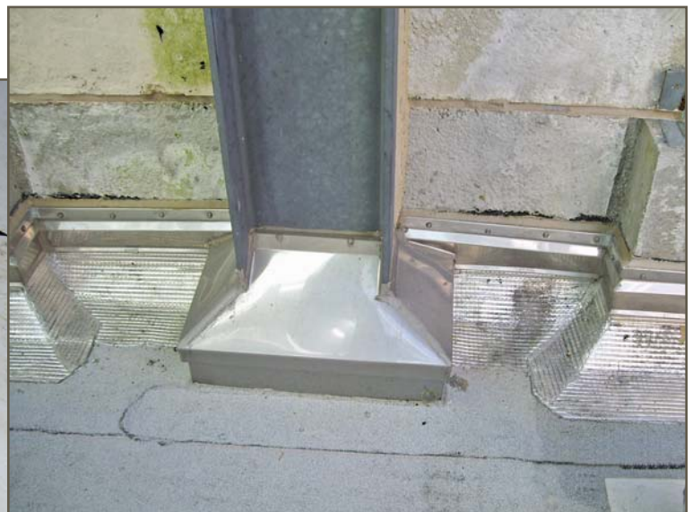
Figure 7 – Sheet metal bonnet installed at I-beam.
