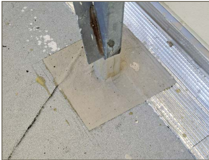
Figure 9 – Liquid flashing membrane installed at steel support.
