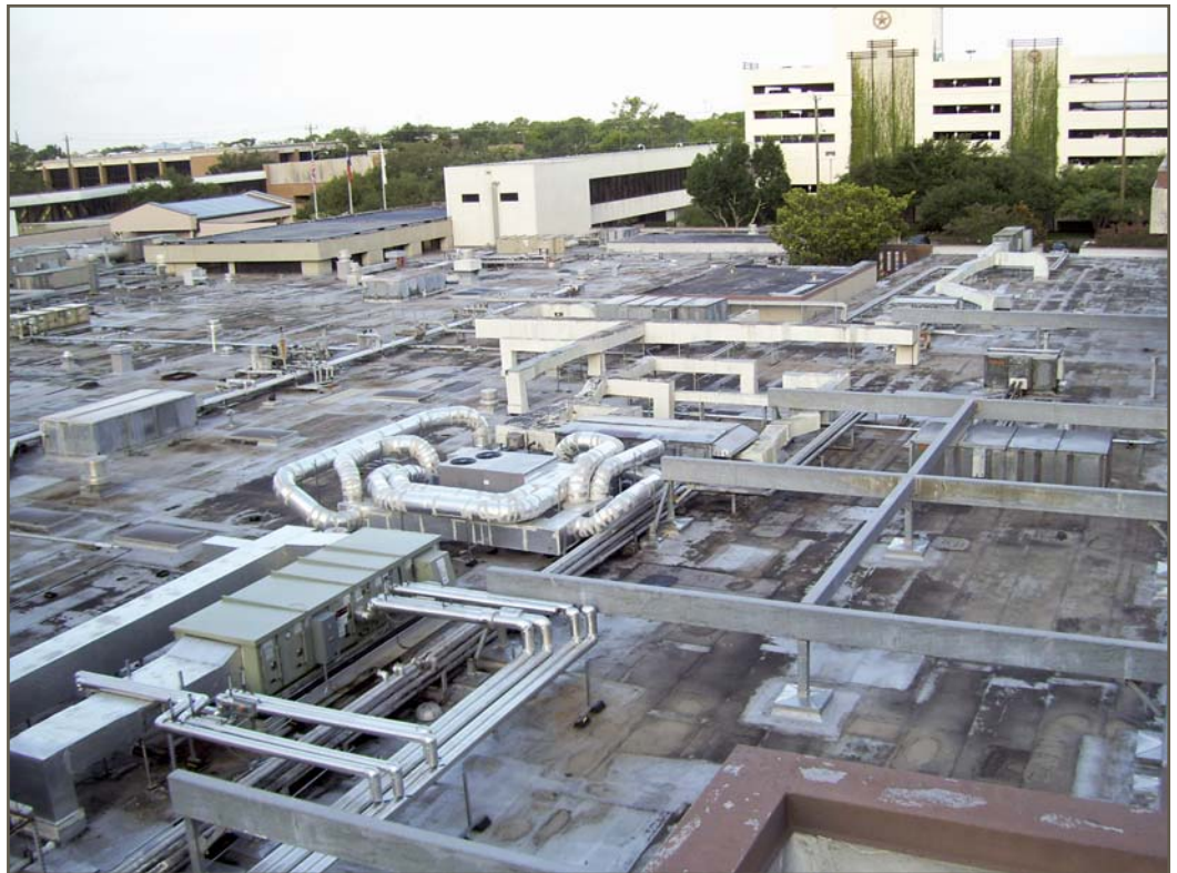
Figure 1 – Overview of rooftop equipment.
