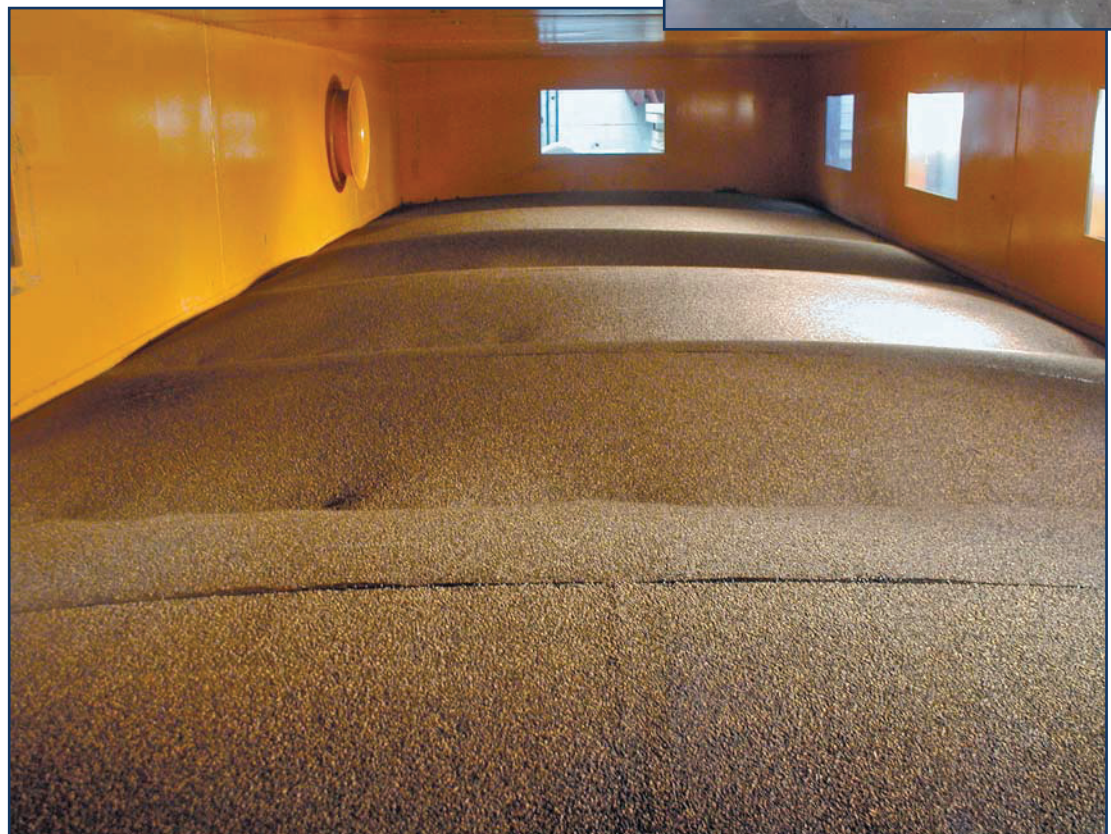
Figure 1E – Billowing of mechanically attached mod bit membrane in the lab.
