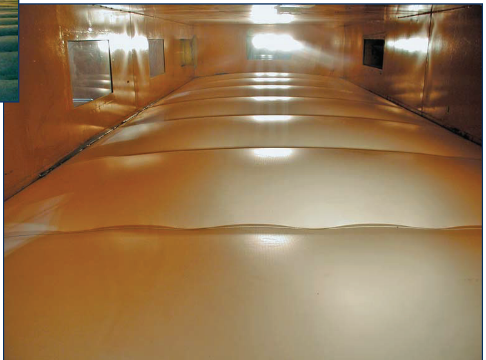
Figure 1B – Billowing of mechanically attached TPO membrane in the lab.
