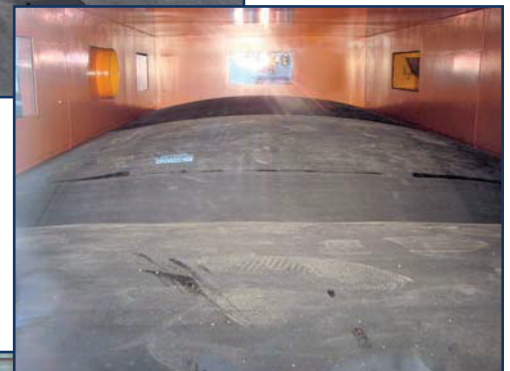
Figure 1D – Billowing of mechanically attached EPDM membrane in the lab.
