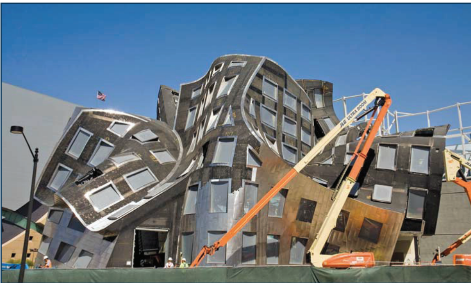
Figure 9 – The Lou Ruvo Center, opened in July 2009, shown here under construction.
