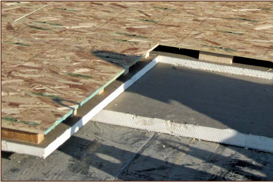
Figure 2 – A typical ventilated nail base.
