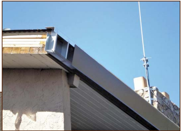
Figure 4 – The vented fascia integrates with the vented nail base to provide airflow for the roof system.
