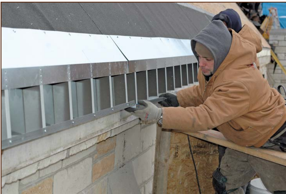
Figure 11 – Installation of the eave ventilation system on St. John’s Lutheran Church.
