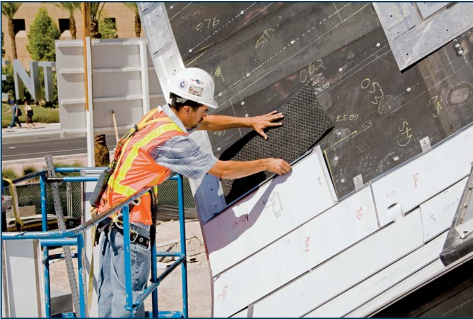
Figure 8 – Installation of an underlayment with incorporated structural separation layer under stainless steel panels at the Cleveland Clinic Lou Ruvo Center for Brain Health in Las Vegas, NV.
