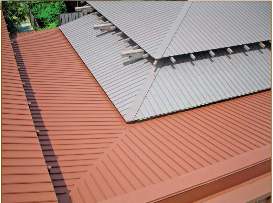
Photos 4A and 4B – This metal roof at Disney World was first detailed with a stable rust primer and foundation coat (left) and then finished with a water-based fluoropolymer coating product (below). The original red color was restored with a color-stable, biologically resistant, “cool color” infrared reflective (IRR) roof. (Photographs courtesy of Quest Construction Products: United Coatings, Spokane, WA.)
