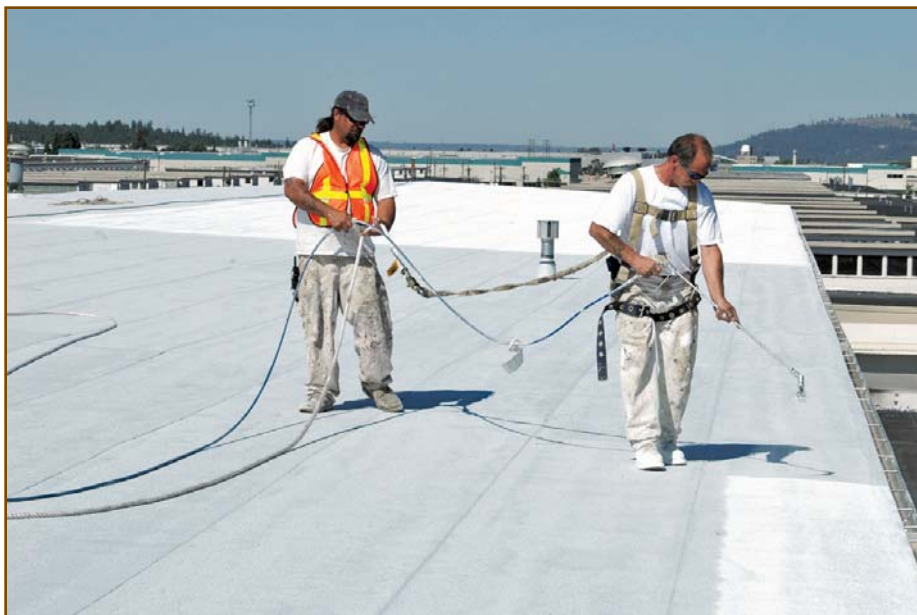
Photo 1 – A specialized gray base coat on this modified-bitumen roofing system blocks asphalt from bleeding into the bright white acrylic topcoat. (Photograph courtesy of Quest Construction Products: United Coatings, Spokane, WA.)
