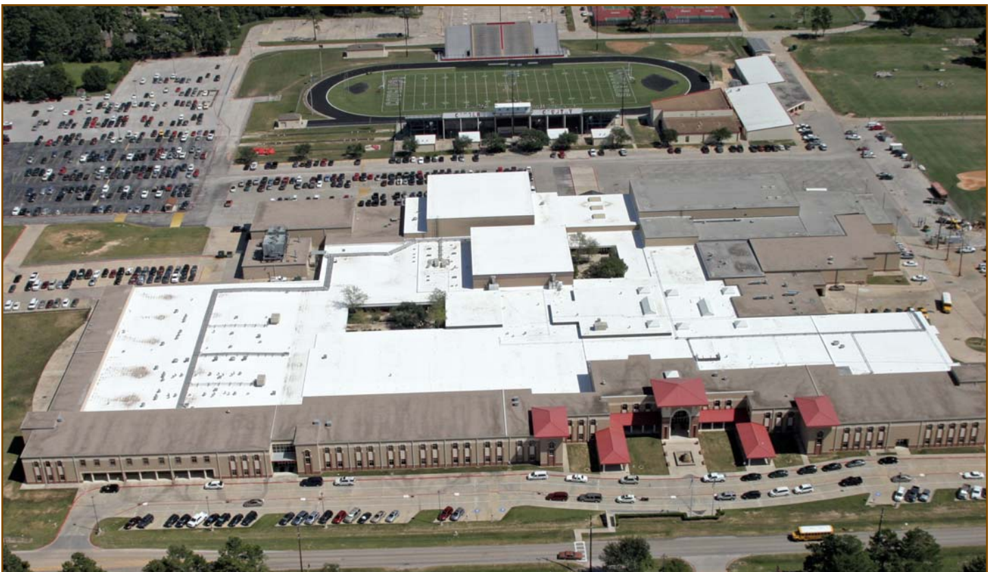
Photo 3 – A monolithic acrylic coating system on this school in Texas provides waterproofing as well as reflectivity and energy savings. (Photograph courtesy of Quest Construction Products: United Coatings, Spokane, WA.)
