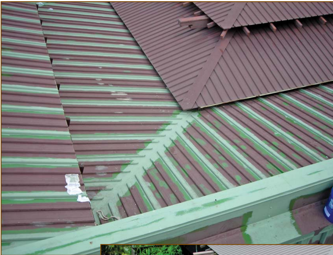
Photos 4A and 4B – This metal roof at Disney World was first detailed with a stable rust primer and foundation coat (left) and then finished with a water-based fluoropolymer coating product (below). The original red color was restored with a color-stable, biologically resistant, “cool color” infrared reflective (IRR) roof. (Photographs courtesy of Quest Construction Products: United Coatings, Spokane, WA.)
