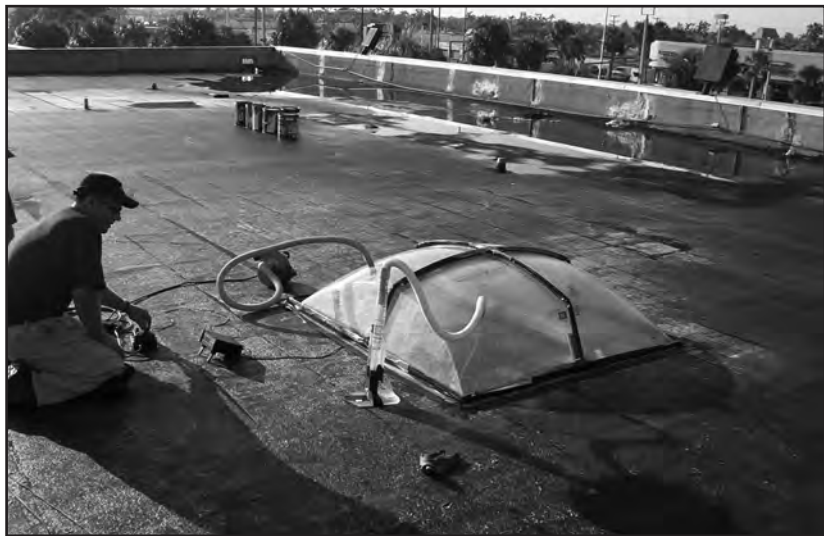
Figure 8 – View of uplift test in progress.
