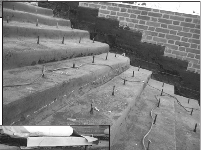
Photo 16 – Uncut protection board lapped over entire portion of stairs. Note that the protection board bulges at stair risers and does not conform to the shape of the stairs.
