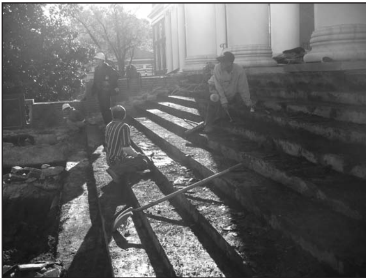
Photo 2 – Removal of existing waterproofing membrane on stairs using handheld-scrappers.
