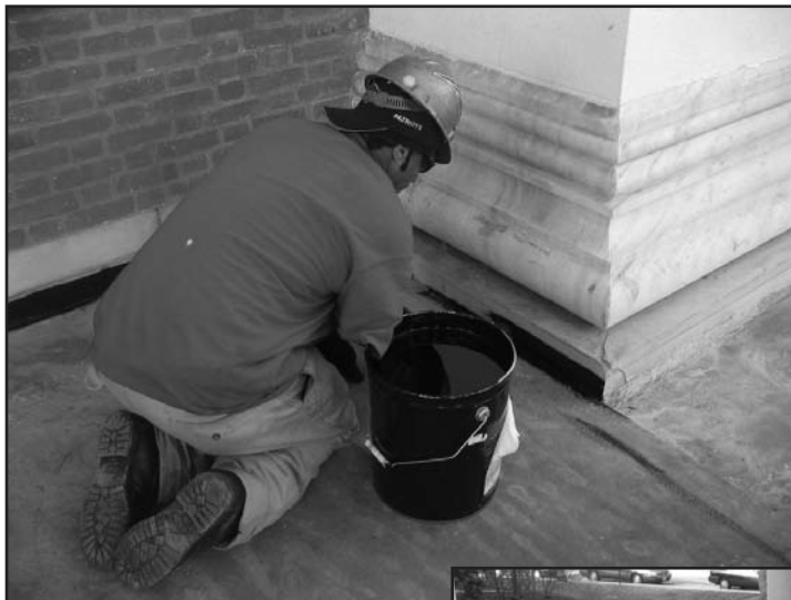
Photo 6 – Primer application with a brush.
