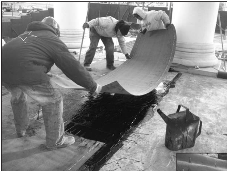
Photo 15 – Placement of protection board over reinforced hot-fluid-applied, rubberized asphalt membrane.
