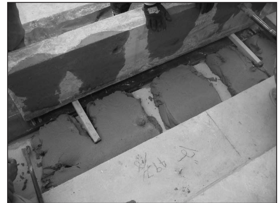
Photo 20 – Alternating mortar-setting beds and drainage space installed below limestone stair treads.
