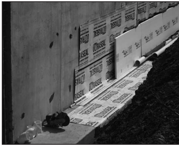
Photo 2 – Installation of a positive-side waterproofing system.
