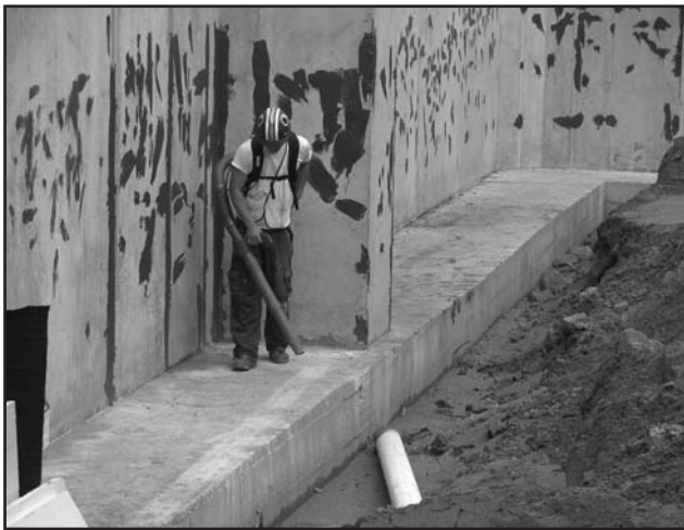
Photo 5 – Preparation of substrate by blowing debris from concrete footing.
