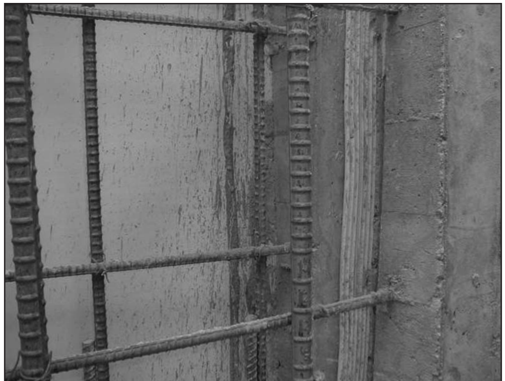
Photo 4 – Ribbed polyvinyl chloride (PVC) waterstop embedded in concrete.
