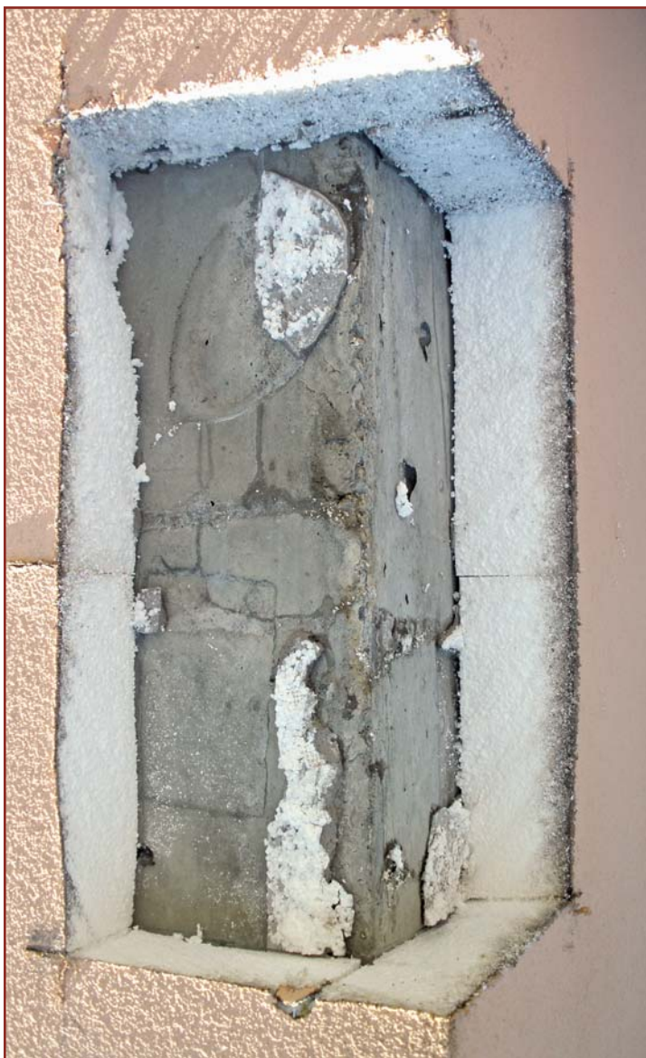
Photo 1 – Test opening at EIFS-clad wall.
