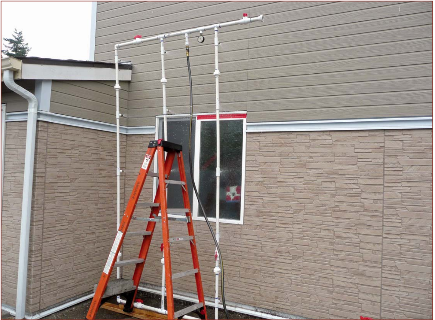
Photo 2 – Field testing of suspect window installation.
