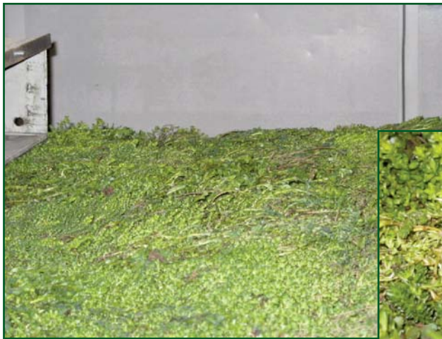
Photo 6 – Sedum planting after two hours' exposure to 110-mph wind. (Photo courtesy of DLR Consultants.)
