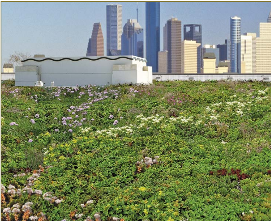
SPRI and the Dept. of Energy have jointly funded a program to quantify the energy savings associated with various types of vegetated roof systems. (Photo courtesy of GAF Materials Corporation, Wayne, NJ.)
