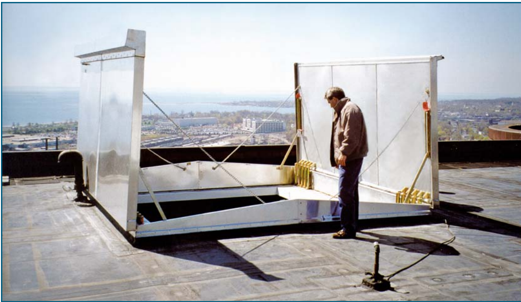
Photo 2 – Equipment-access roof hatches serve as a means of entry for large pieces of equipment and are generally double-cover models that are custom-manufactured to specific size requirements.
