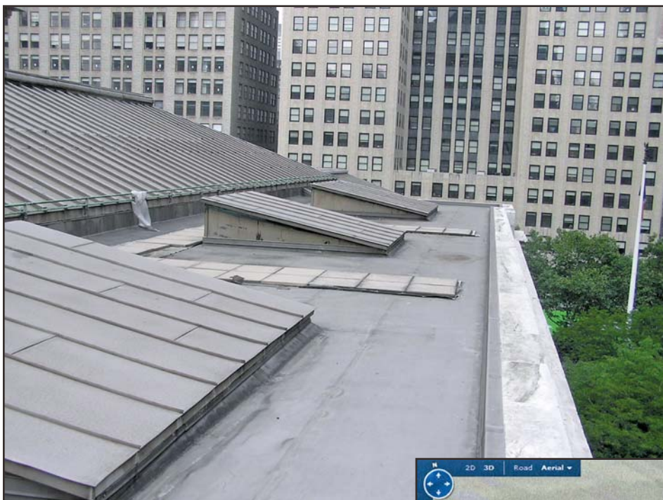
Photo 7 – Photo taken from the roof above the 5th Avenue entrance to the library.
